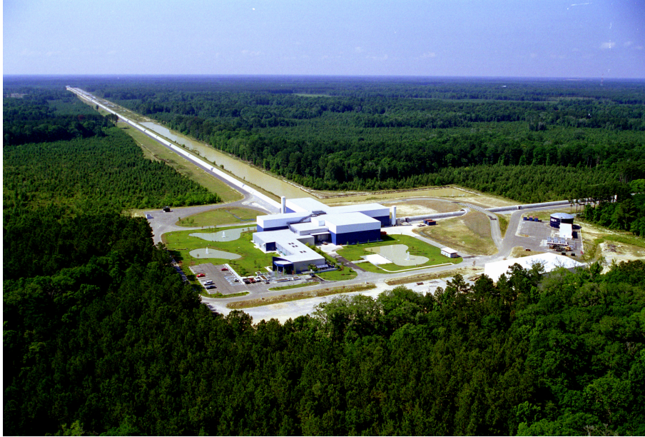
Figure 10. Aerial view of the LIGO Livingston Observatory. The protective covers over the vacuum tubes indicate the light path from the corner station (with laser and beamsplitter) to the end interferometer arm mirrors 4km distant. Reports on Progress in Physics , v.72 (2009)
