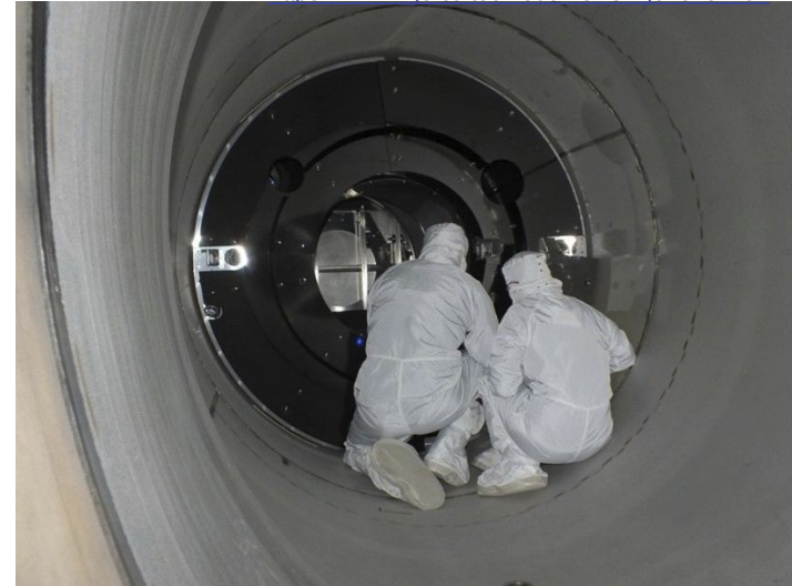
DLC coated SSTL baffle installation
