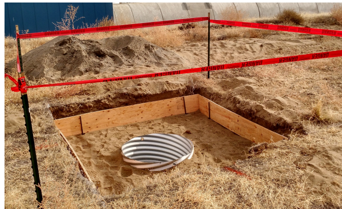
Hole for one of H1 wind-fence posts.
