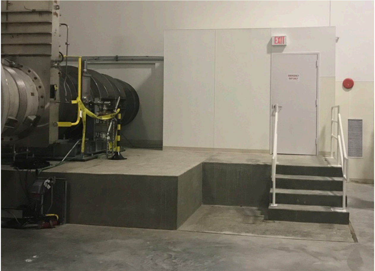
Figure 8: Livingston LVEA +Y wall. Main Y beamtube is shown at left as it enters the BTE (Figure 6). New FC tube penetration may intersect the existing exit door, pictured at right. Access door into new FCTE is required to the left of this. Top of raised concrete slab is approximate BTE and new FCTE floor level.
