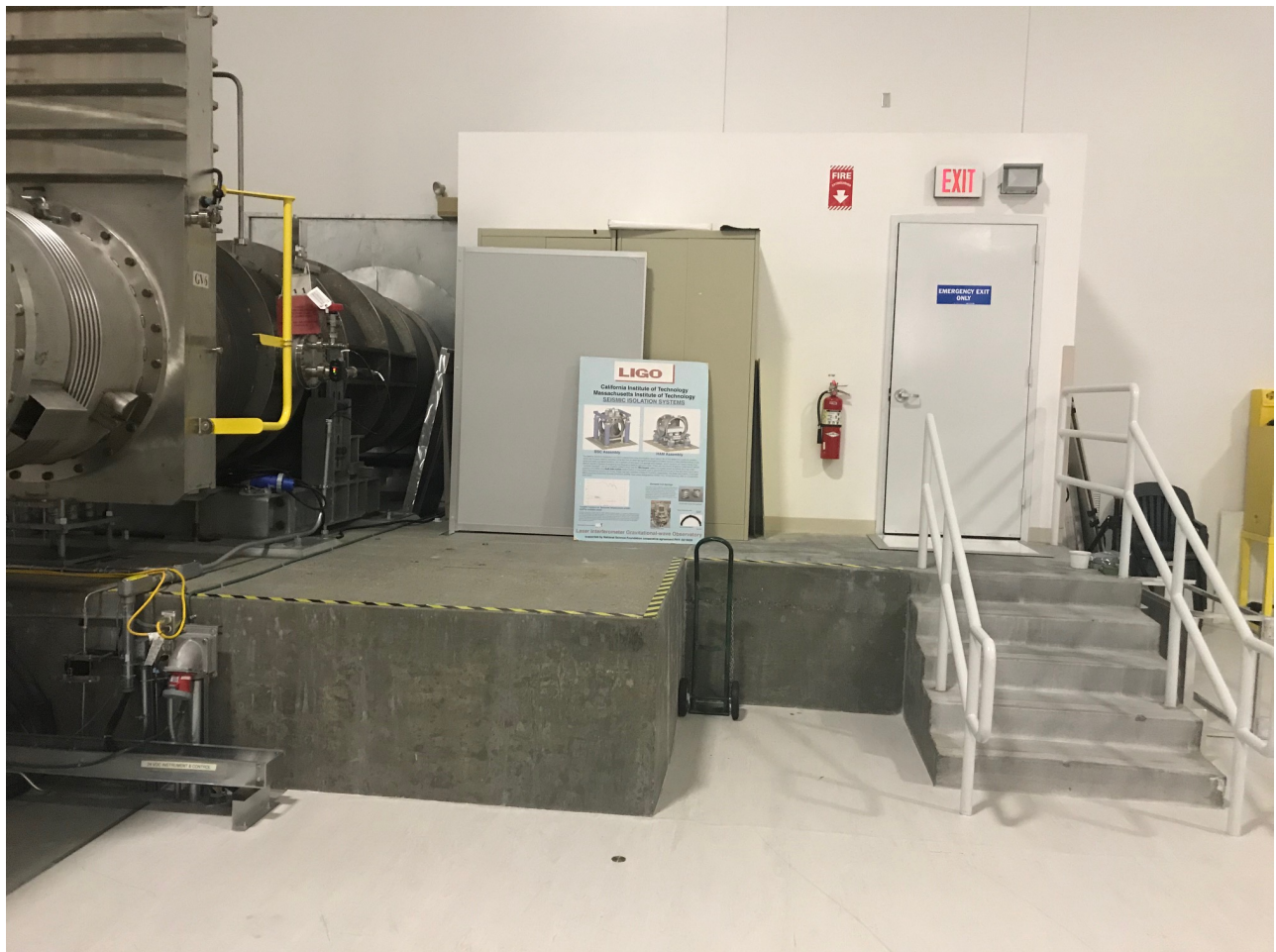
Figure 7: Hanford LVEA +Y wall. Main Y beamtube is shown at left where it enters the BTE (Figure 6). New FC tube penetration intersects the existing exit door pictured at right. Access
