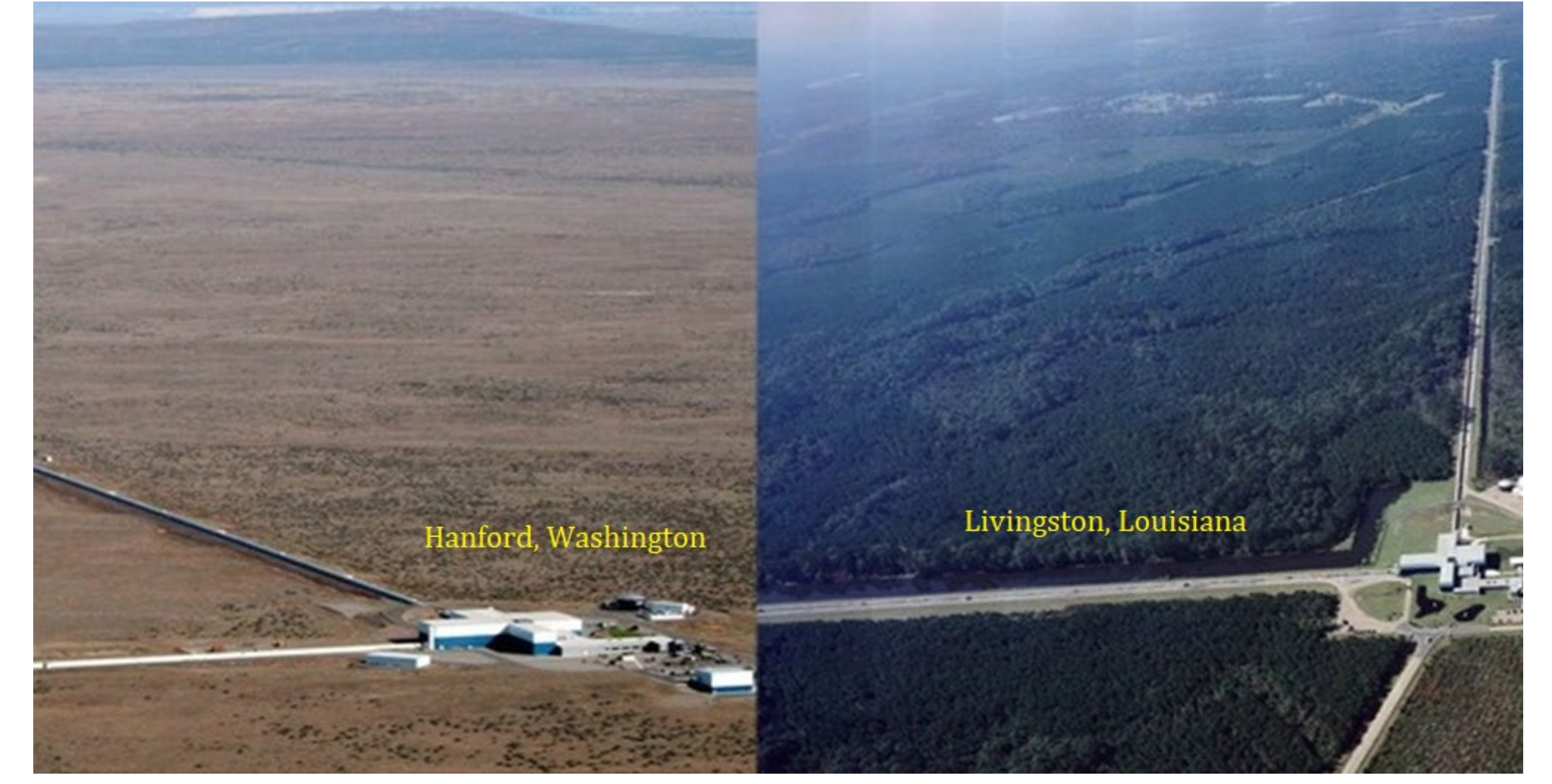
Two aerial photos of the two largest LIGO detectors, each sending a laser down a 4km vacuum chamber with mirrors at each end. The mirrors multiply the path length of the laser, transforming the 4km cavity to one that is effectively 1120km.
