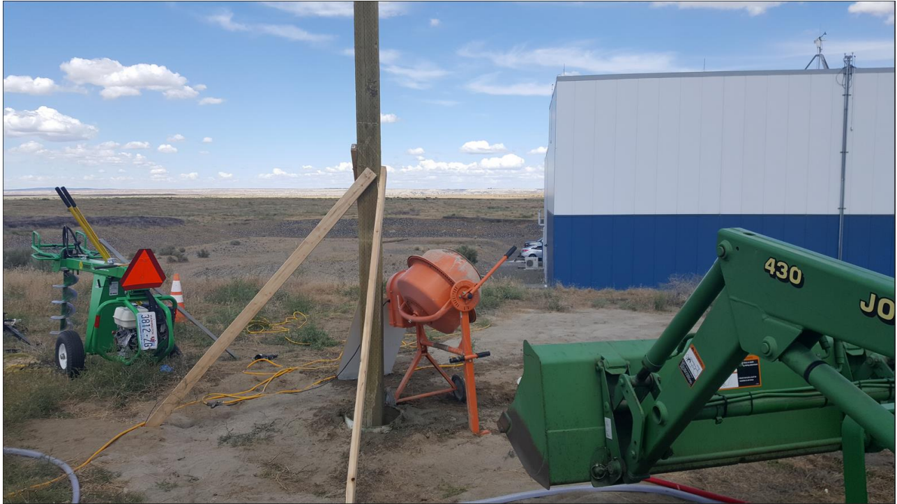
Figure 15: Setting a Post for Prototype Wind Fence
