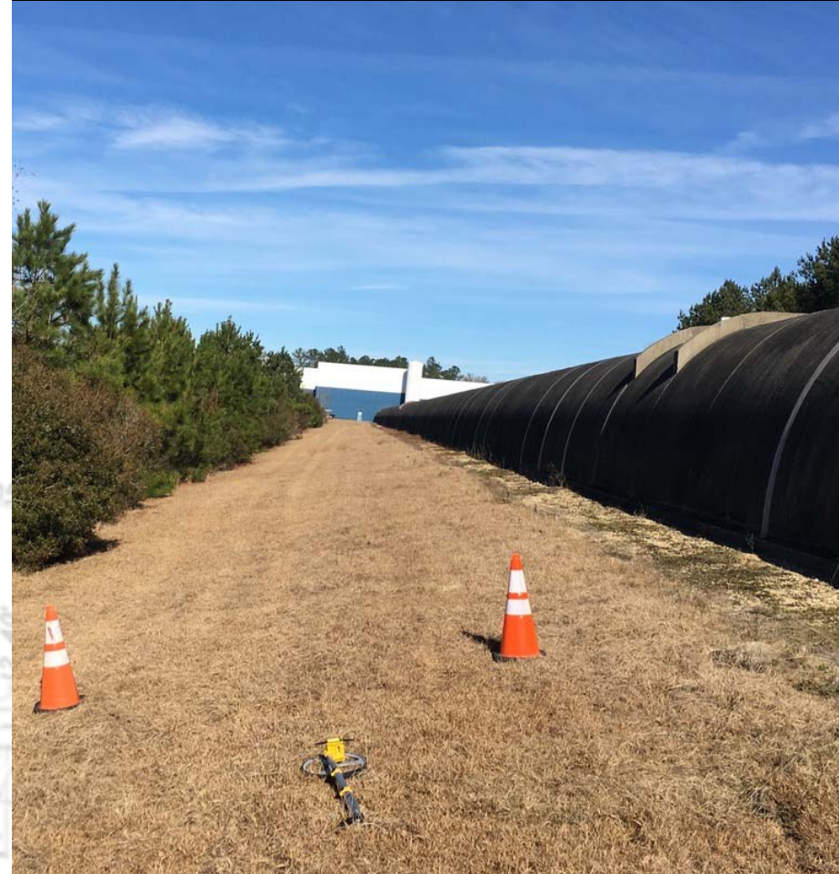
View from future LLO FC end station back to corner
