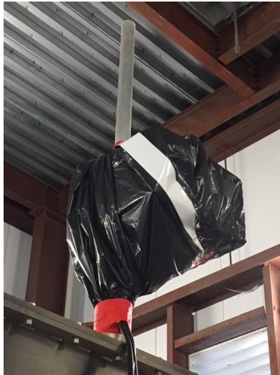
Figure 2: Bag encapsulating GV8 actuator mechanism on 10/19/17. Argon was admitted through a 1/4" Polyflo tube laid alongside the electrical cables at bottom. The end followed the cables into the rectangular motor housing.
