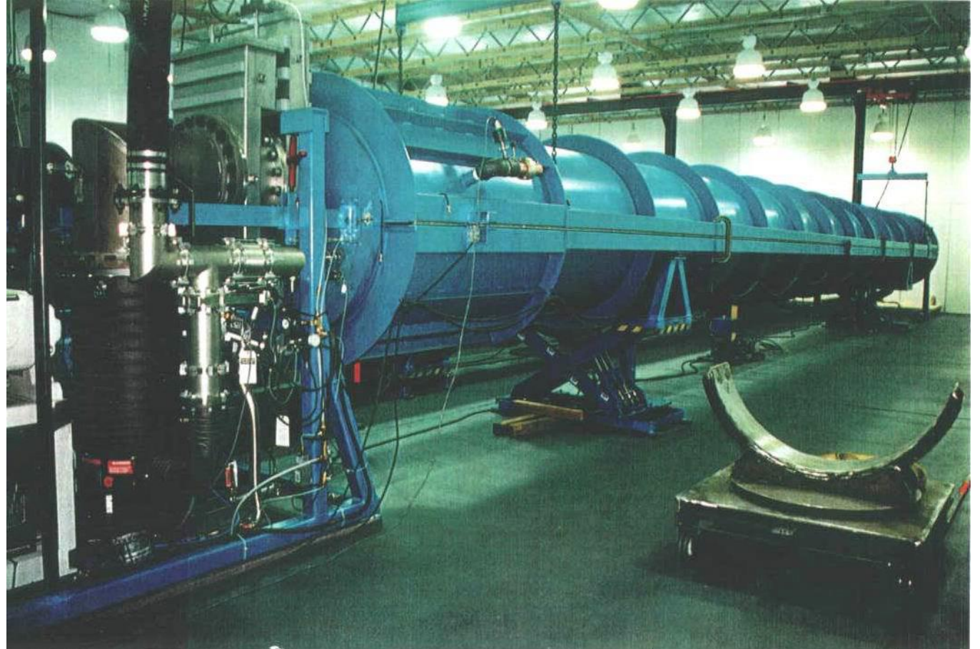
Helium leak testing a section of beam tube. Note large diffusion pump, Roots-backed forepump
