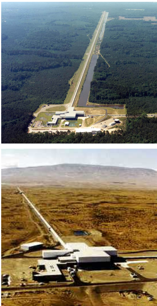
FIG. 4. Images showing the two LIGO sites in Livingston, Louisiana (top) and Hanford, Washington (bottom). The interferometer arms in each detector are 4 km long and contain vacuum pipes along the whole optical path.
