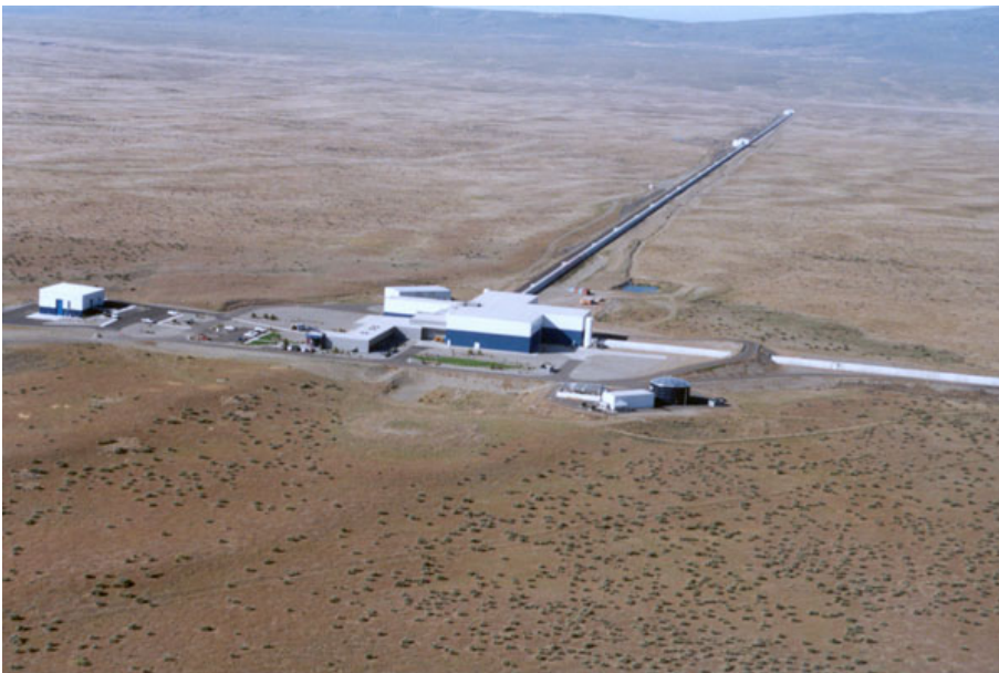
Figure 3.2: An arial view of LIGO Hanford (H1 and H2) showing the full y-arm, part of the x-arm and the exterior building around the control room and laser and vacuum equipment area. Image taken from www.ligo.org .
