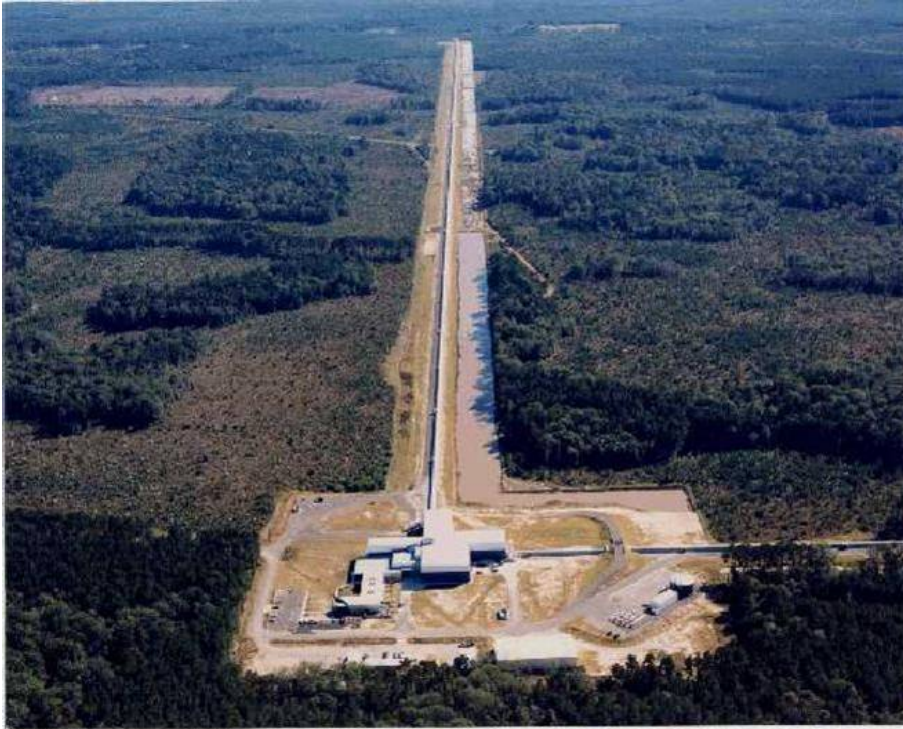
Figure 3.1: An arial view of LIGO Livingston (L1) showing the full y-arm, part of the x-arm and the exterior building around the control room and laser and vacuum equipment area. Image taken from www.ligo.org .
