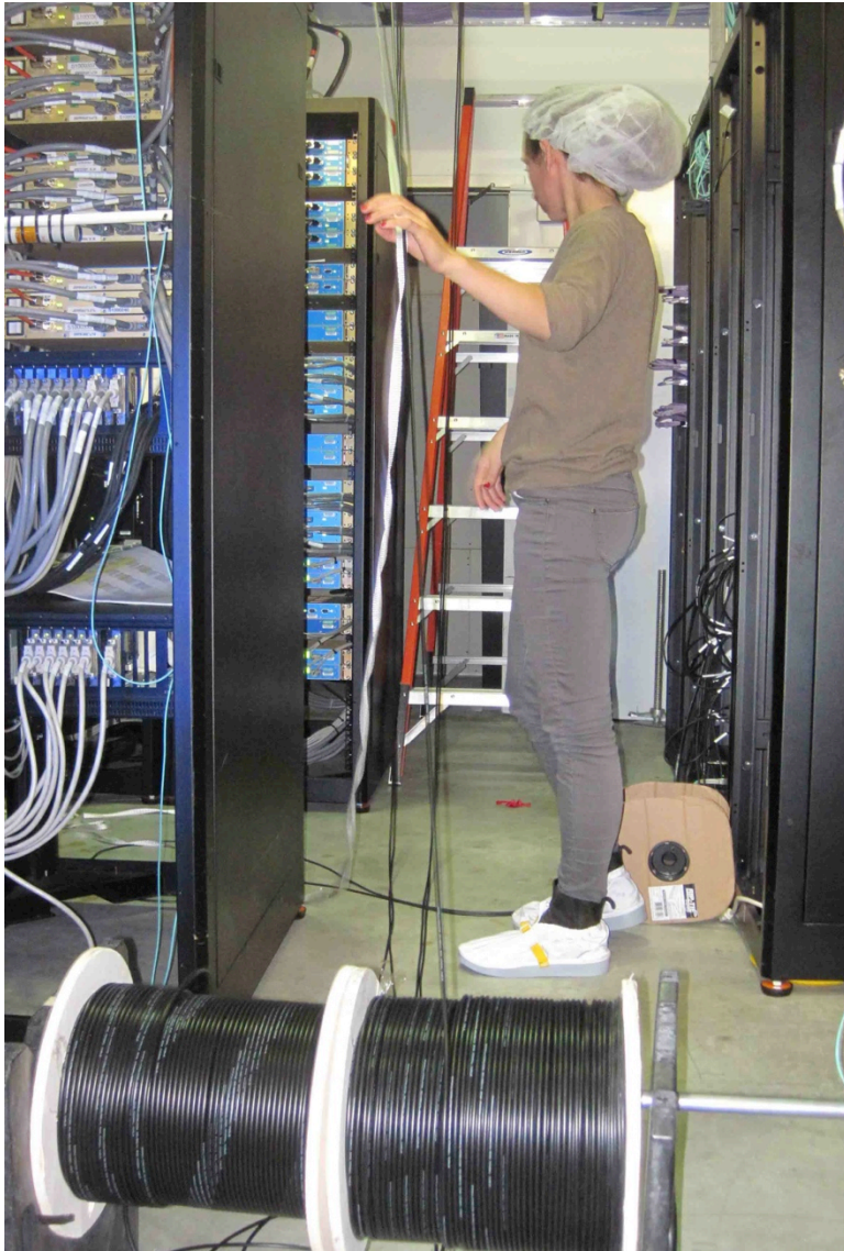
Terra pulling and guiding in e-bay
