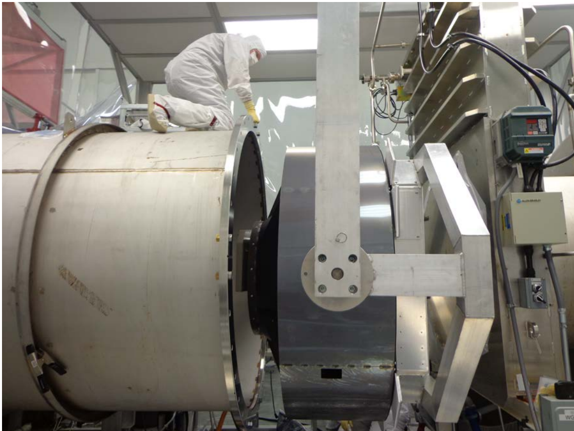
Figure 34: Baffle between spool and gate valve
