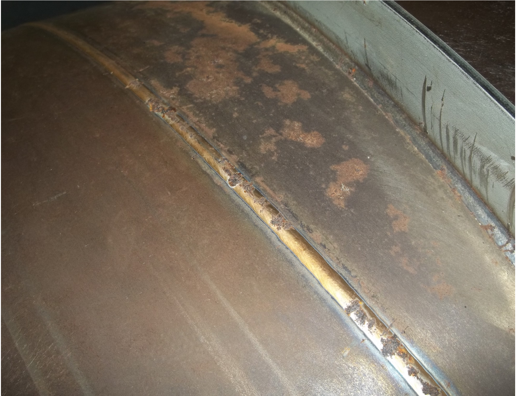
Corrosion on spiral weld, tube and continuous stiffening ring weld
