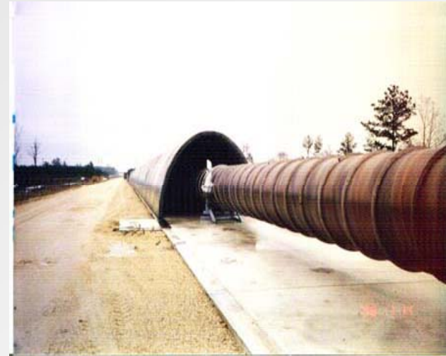
Beam Tubes: 1.2 m diameter - 3mm stainless, 50 km of weld.... and not one leak!
