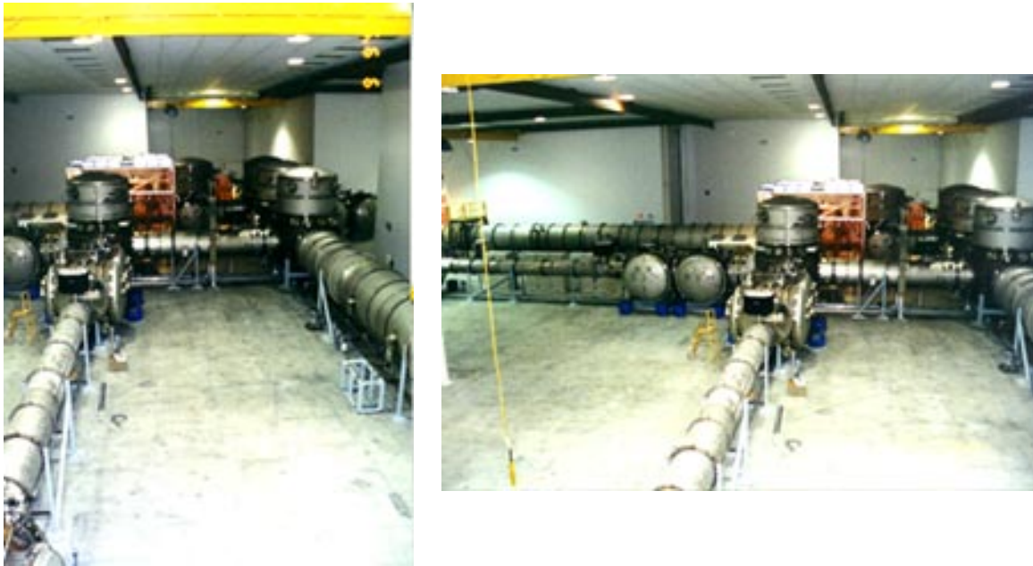
FIGURE 1. Hanford Laser and Vacuum Equipment Area (LVEA).
