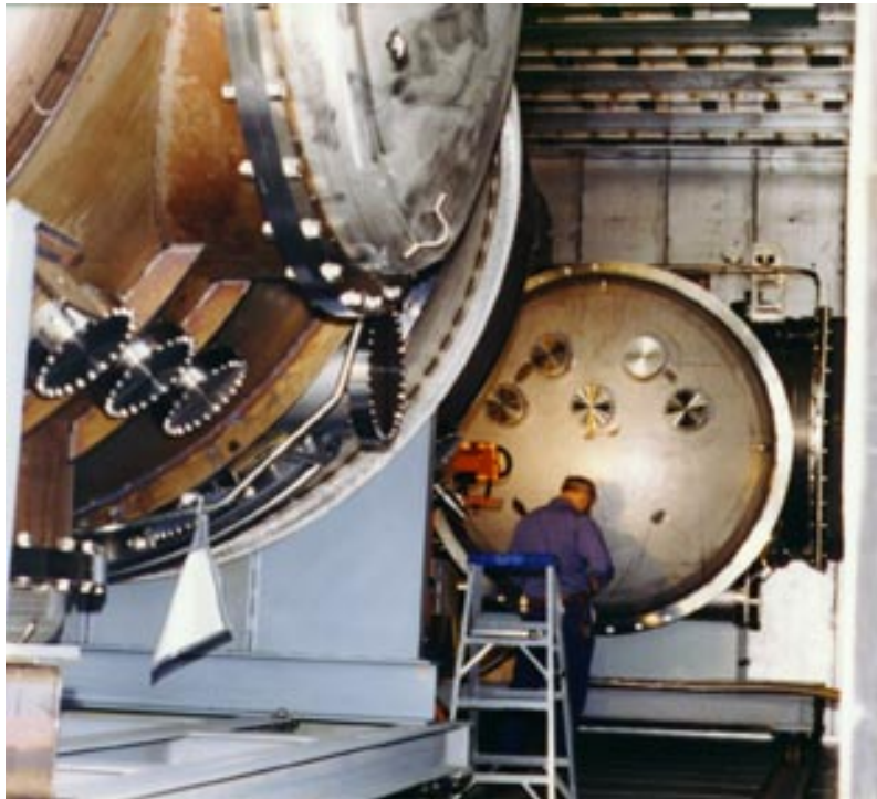
FIGURE 8. Inside the Large Component Bake Oven at PSI.
