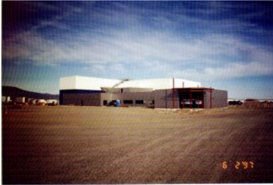
FIGURE 16. The Corner Station from Main Entrance at Hanford Site.
