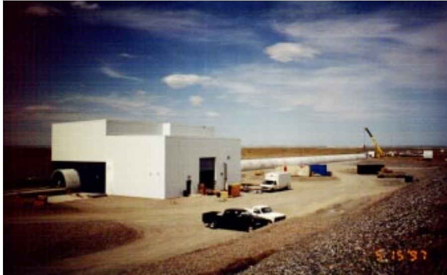
FIGURE 14. Installation of Beam Tube Enclosure Segments along Southwest Arm
