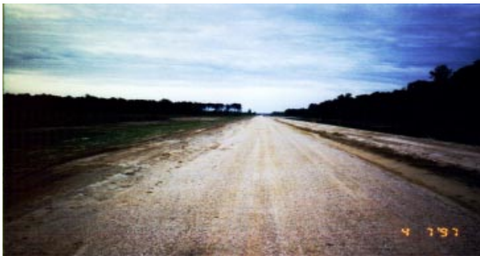
FIGURE 13. View of the Access Road along Southeast Arm at Livingston.
