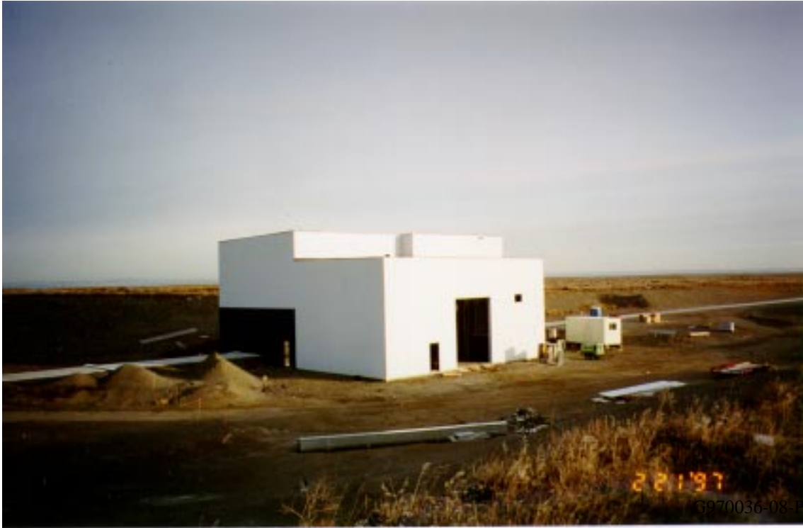
FIGURE 16. View of Mid Station on Southwest Arm at the Hanford Site.
