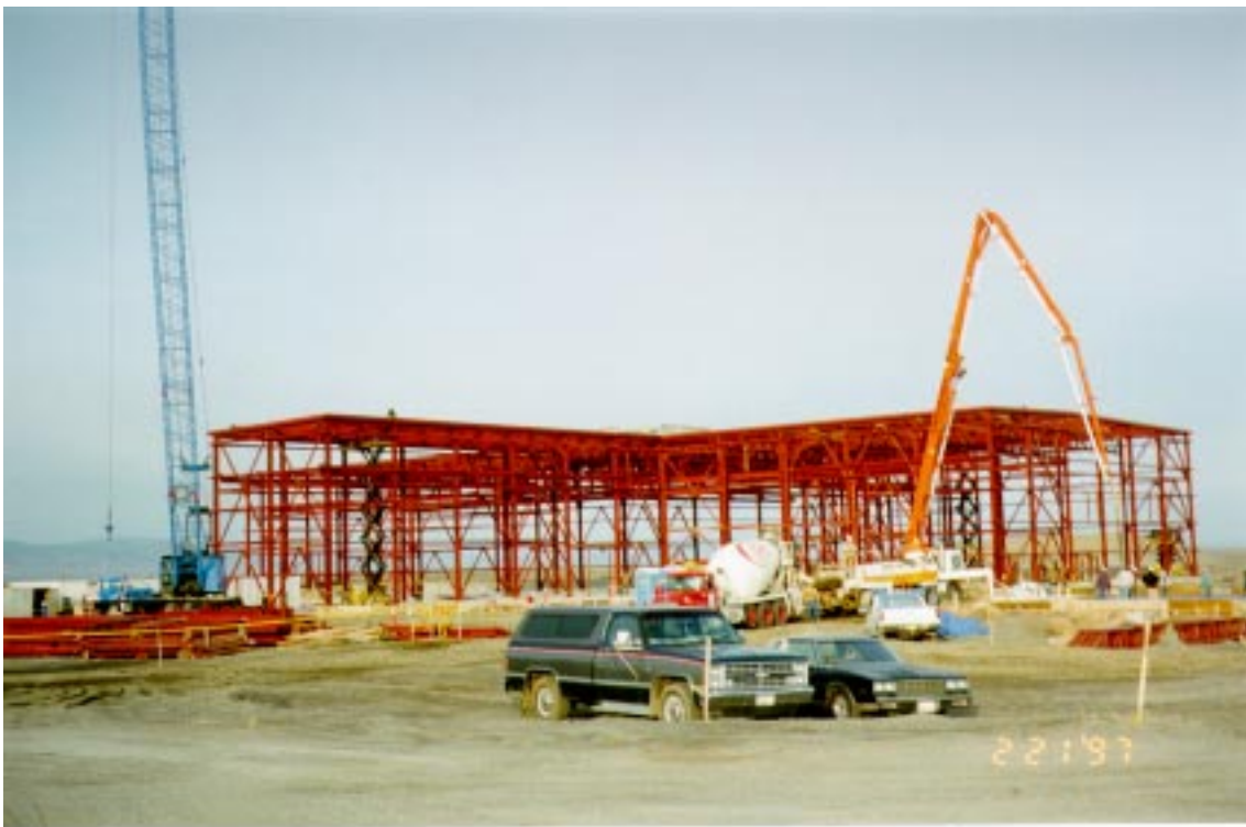
FIGURE 15. View of LVEA at Hanford
