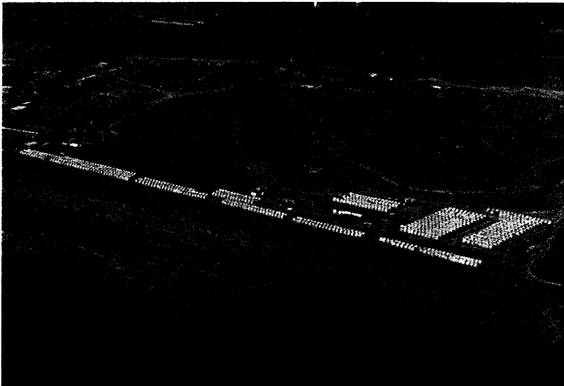
FIGURE 15. Completed Beam Tube Enclosure Segments at Contractor's Site
