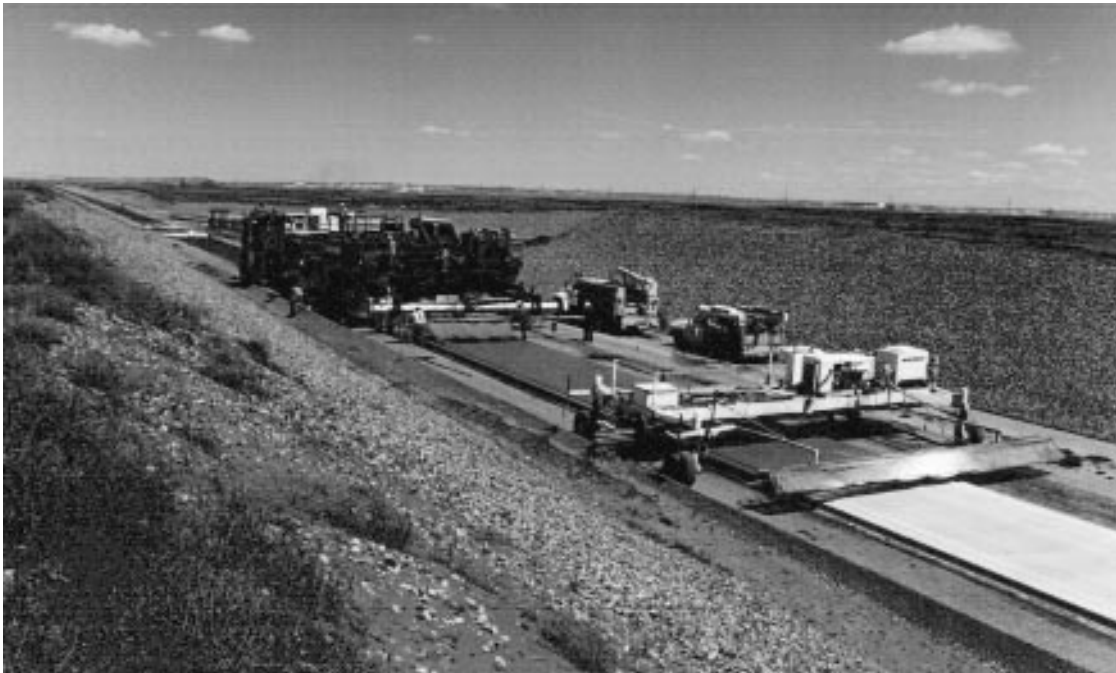
FIGURE 6. Slip-forming and placement of concrete for beam tube enclosure slab
