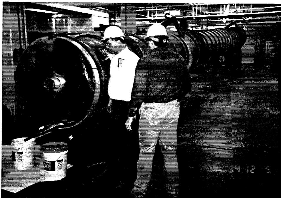
**Draining Mirachem 500 from 22A Beam Tube Assembly**
