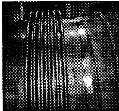
The third circumferential joint was between the expansion joint and assembly 21-D. The expansion joint has a 48.935" inside diameter. The beam tube has a 48.892" outside diameter. The inside offset of .021" and difference in thickness caused concern.
