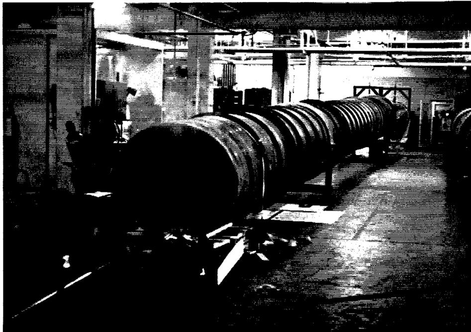
**Steam Cleaning the 22A Beam Tube Assembly per CL1QT**
