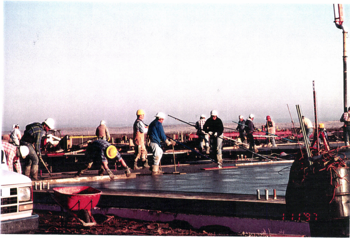
Tamping, screeding, floating and checking tolerance shown here.
