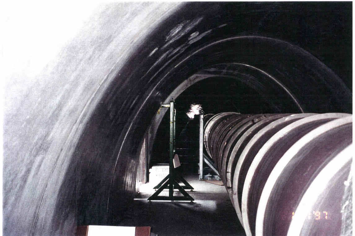
View from the inside of the beam tube enclosure at the Mid Station looking toward the Corner Station.
