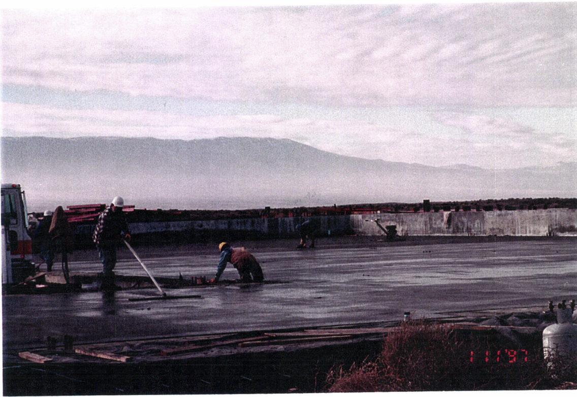
Edge finishing, floating and power troweling continues late into the night.
