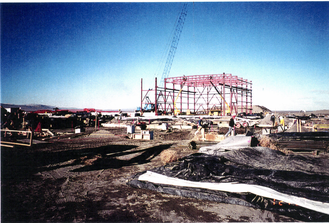
View of the OSB technical support areas. Grading for building slabs continues.
