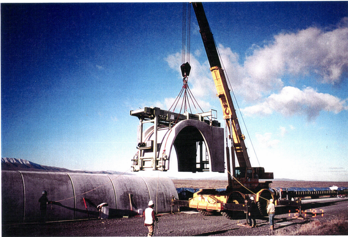
View of the Northwest Arm beam tube enclosure. Setting of the first Type "A" unit.
