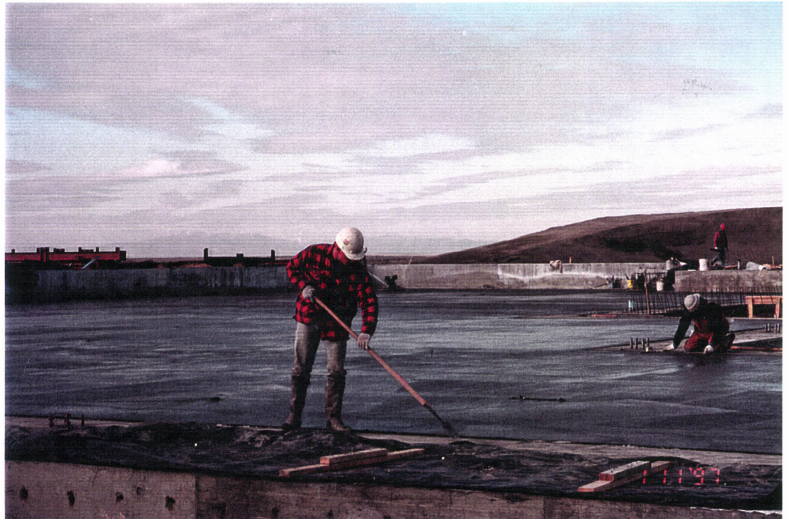
Cleaning up the edges of the grade beam.
