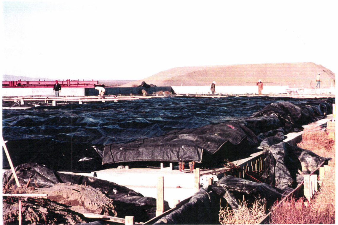
A second cover and heaters were added.
