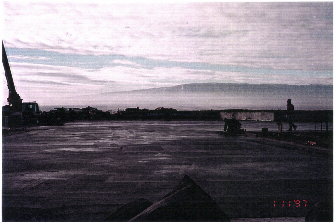
Looking toward the southwest arm of the placed LVEA technical slab.
