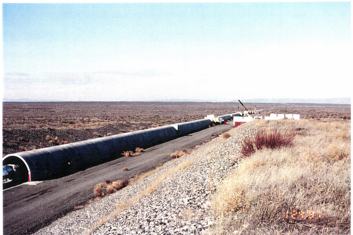
View of the Northwest Arm beam tube enclosure installation. Over 200 BTE's have been installed.
