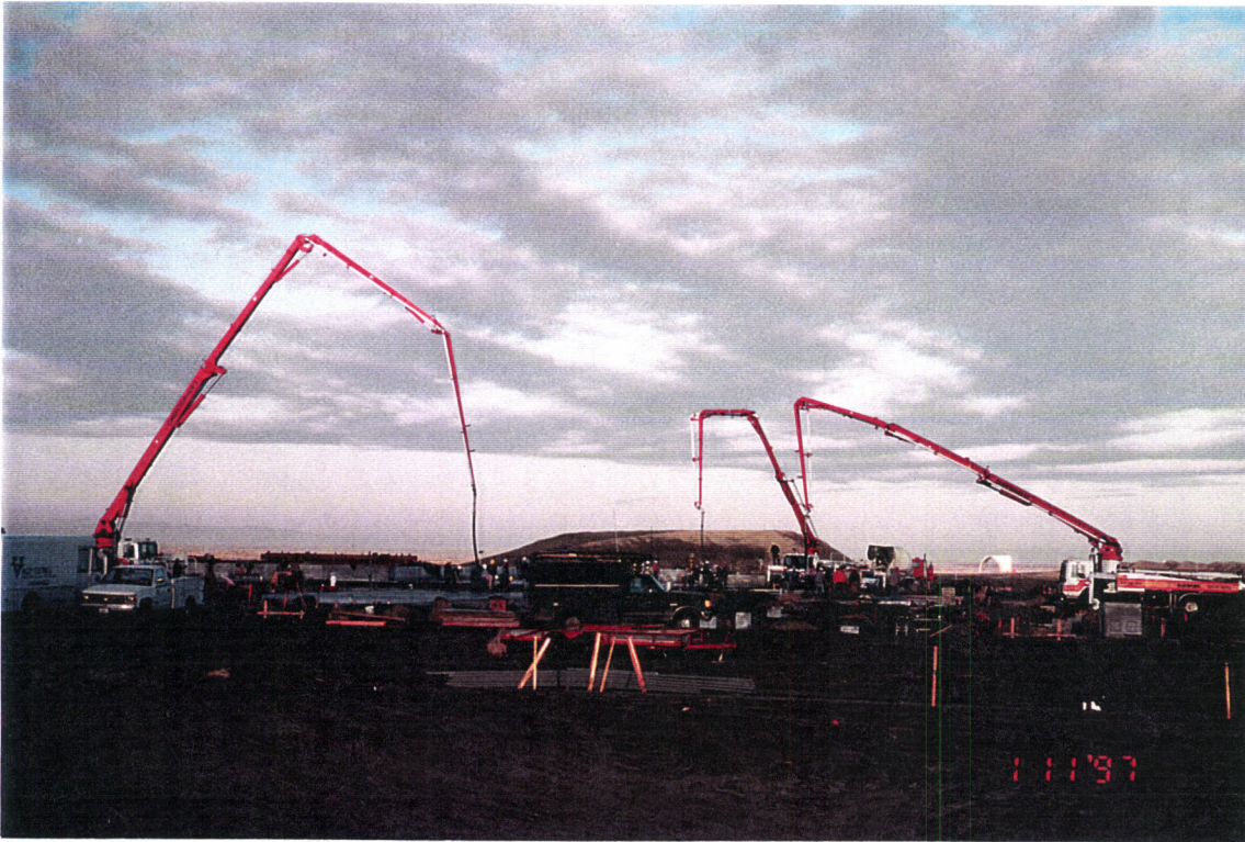
Placing final 6" lift of the Corner Station LVEA. 3 concrete pump trucks were used to place the 500+ yards.
