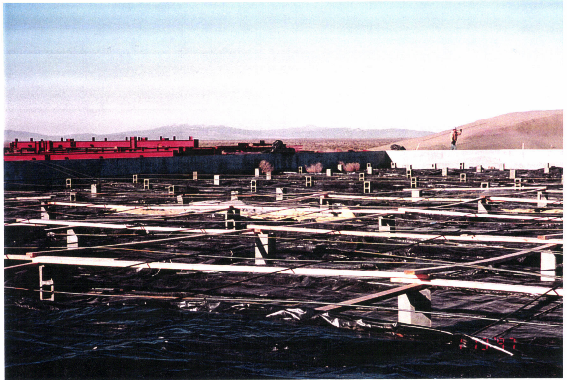
After the first two days extra precaution was taken to protect the slab from freezing.
