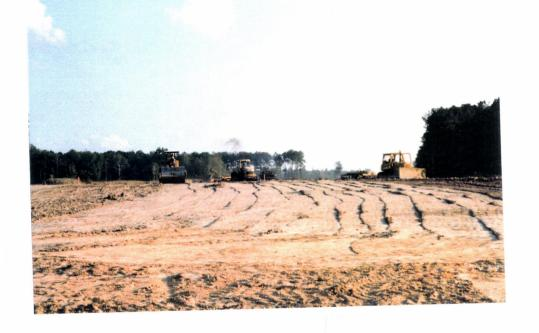
19. Corner station, sealing off fill prior to forecasted rain.
