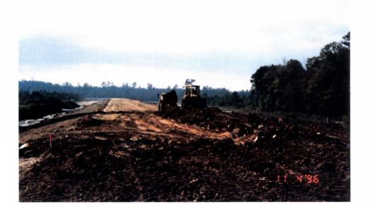
12. Southeast arm, placing fill on berm. G960190- 12. -O-P
