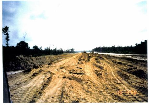
4. Southeast arm at station 36+00 showing a lift of moist material being added. Note truck tire prints assisting in compaction.
