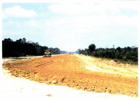
12. Southeast arm at station 132+00 disking a lift of berm.
