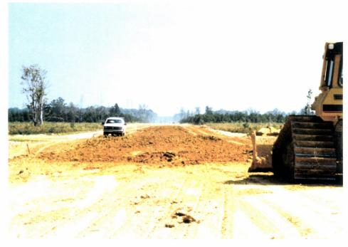
3. Southwest arm at pipeline crossing, adding fill to bring berm up to elevation.
