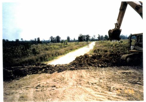
22. Southwest arm at station 98+00. Contractor is building a soil blockade to keep 4x4 activity at a minimum.
