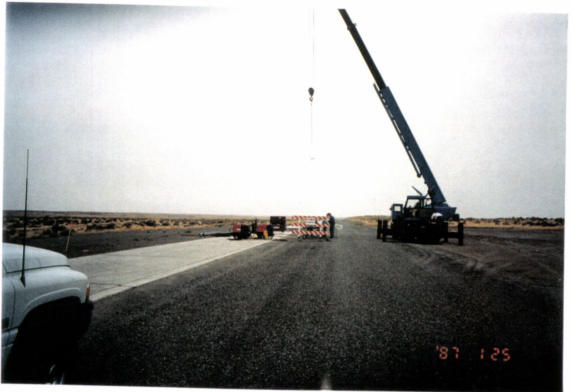
62- CB & I crew set up at the NW mid station.
