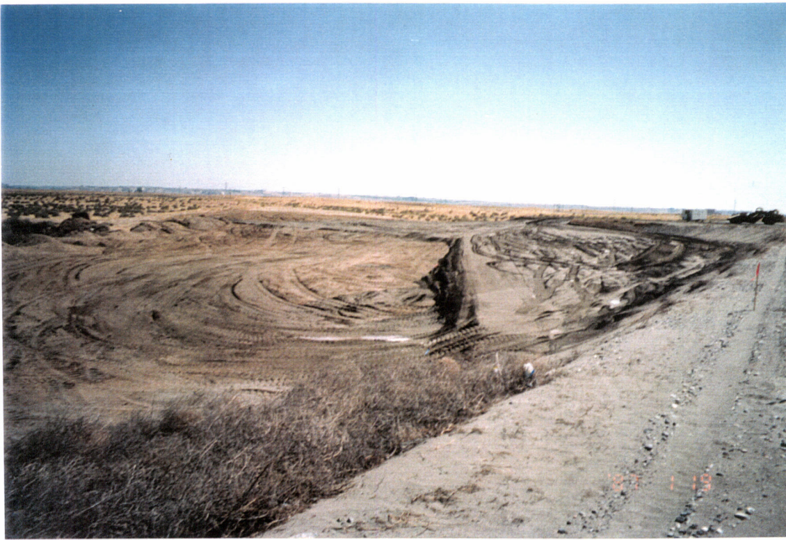
59- Grubbing for chiller pads at the corner station.
