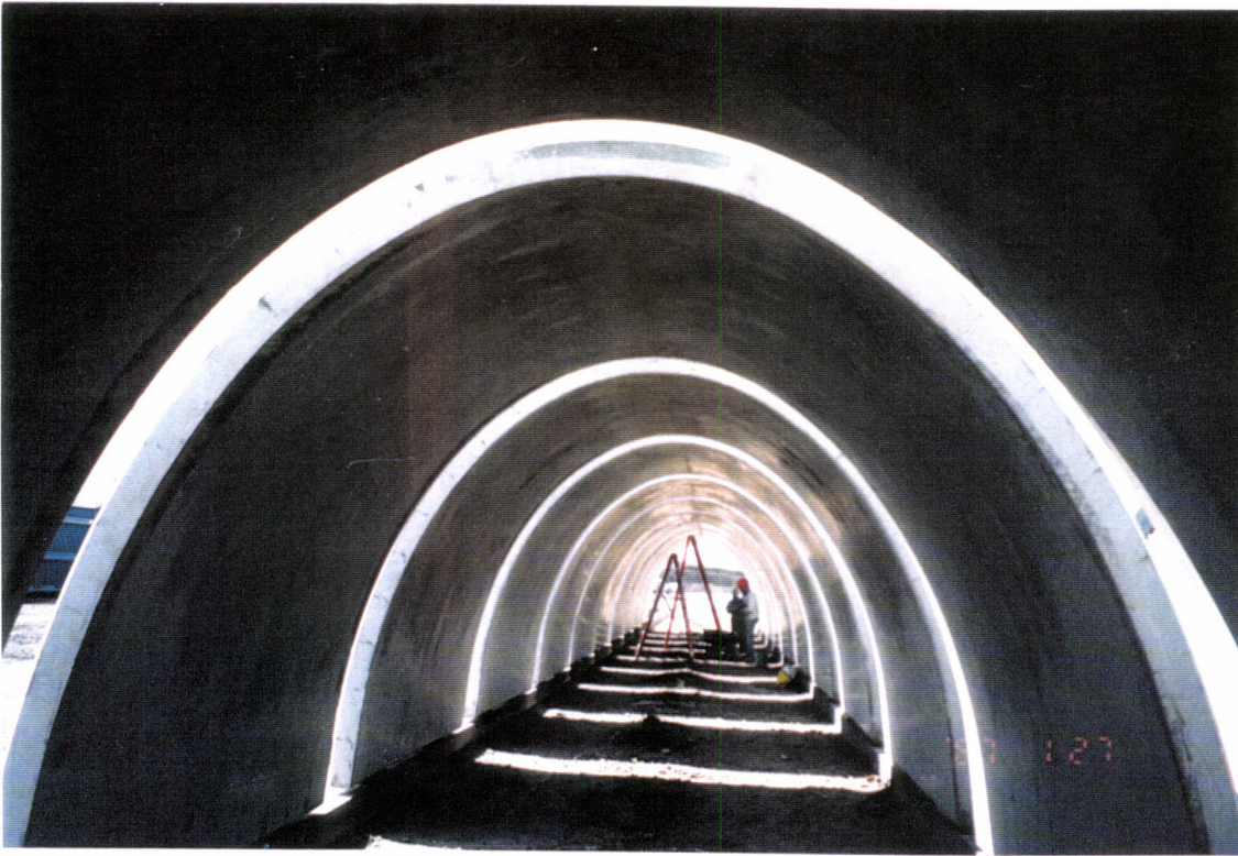
67- An inside view of the Type 'C' enclosures at the Pre cast yard - The workers are doing remedial work.
