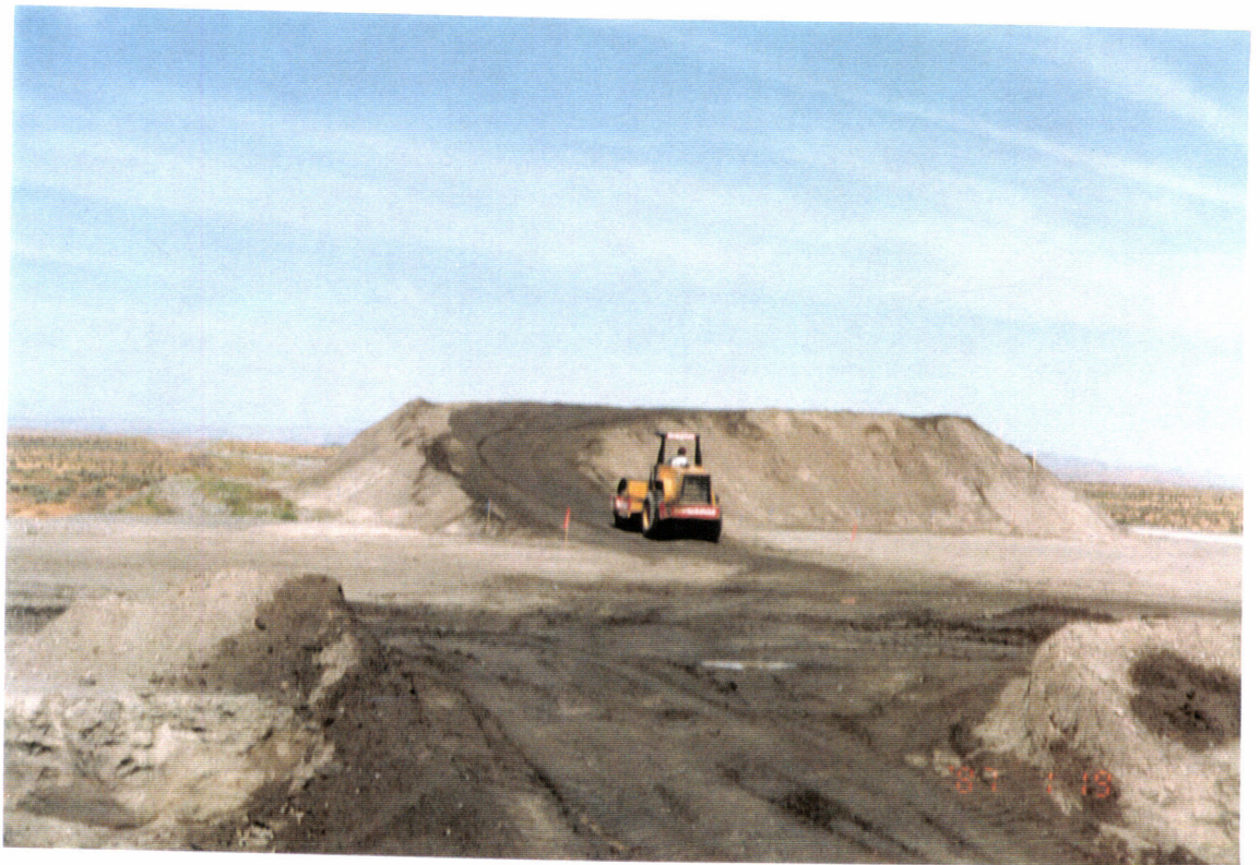
58- Fill for the overpass ramp is being compacted some more.
