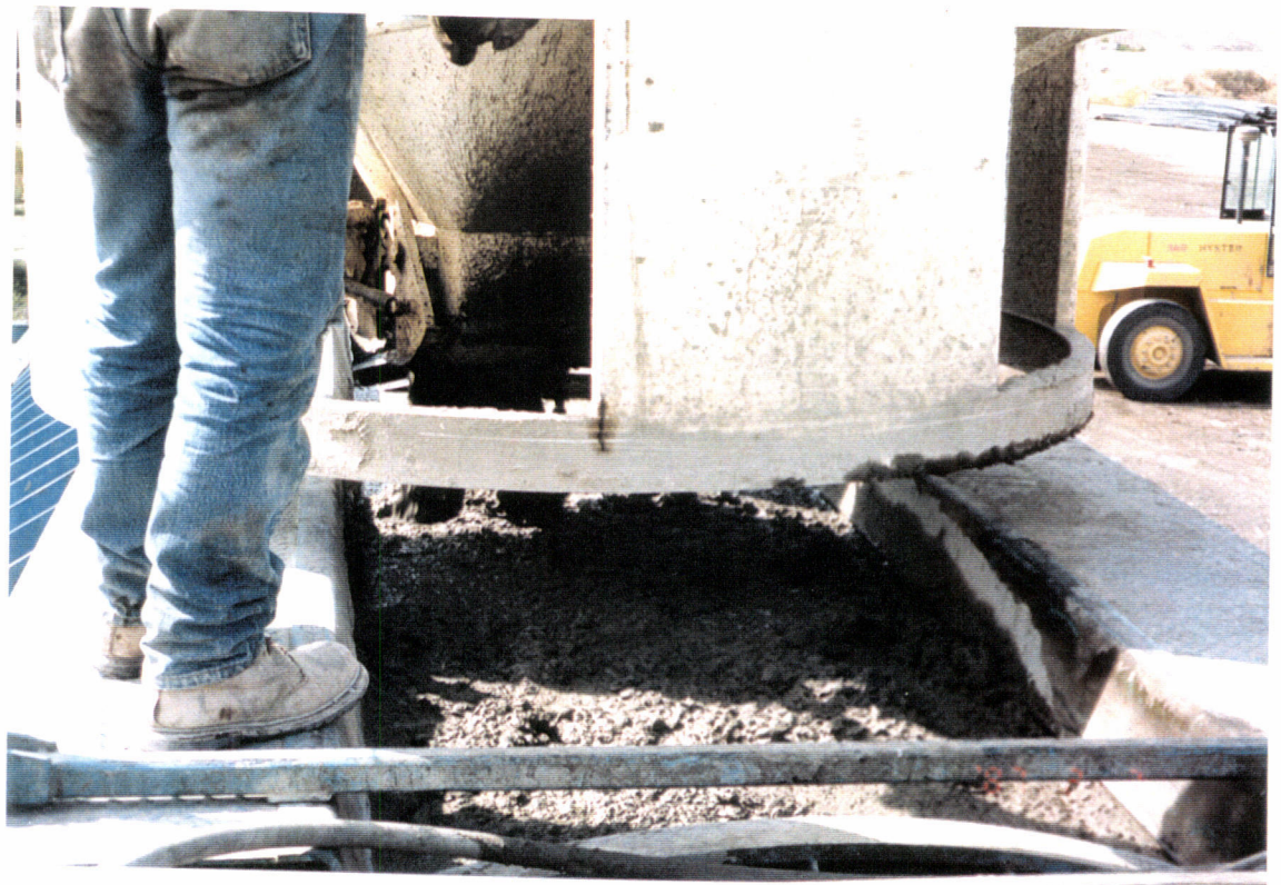
68- Pouring beam tube enclosures at the Pre cast yard.
