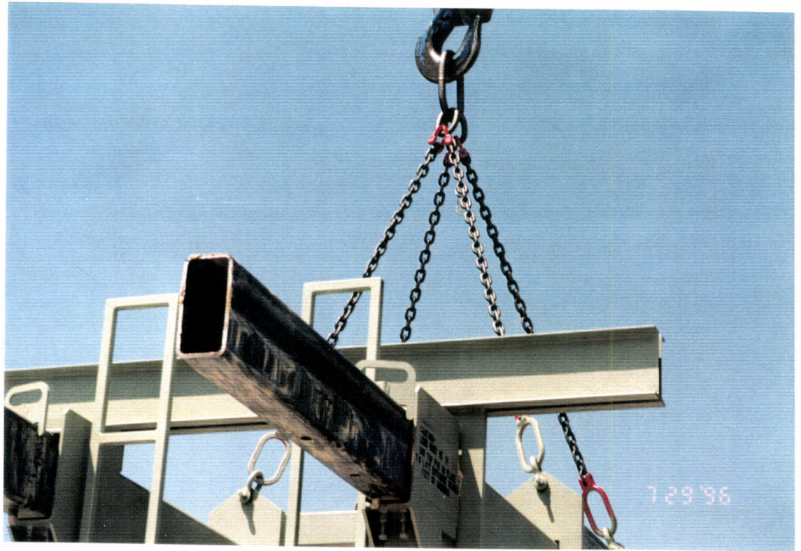
Crane lifting the beam tube enclosure lifting device.
