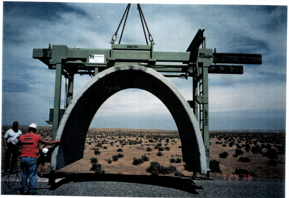
Different view during the lifting and setting of the type "C" beam tube enclosure module.
