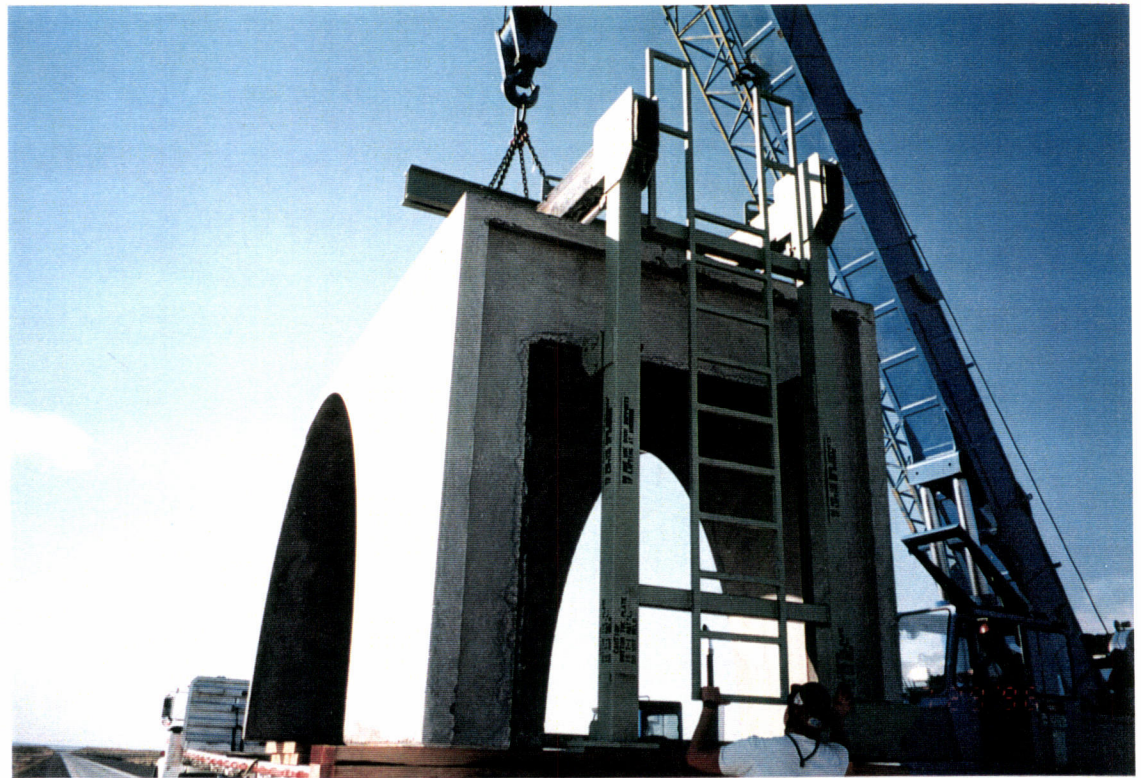
View of the unloading activities for the type "A" beam tube enclosure module.
