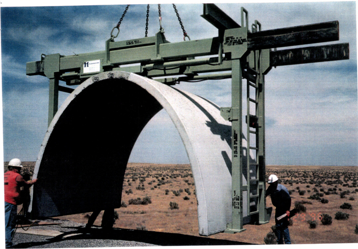
Different view during the lifting and setting of the type "C" beam tube enclosure module.
