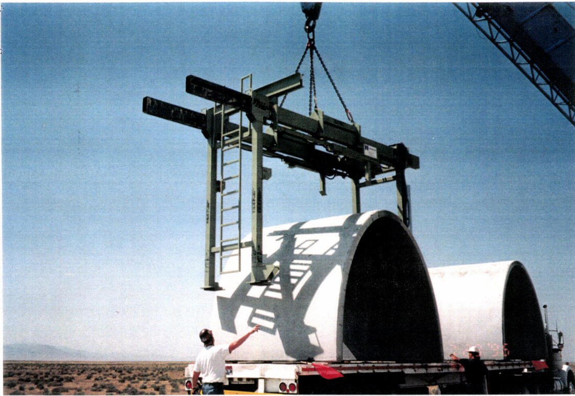
The enclosure lifting device is being aligned to pick the first type "C" module off the delivery truck.
