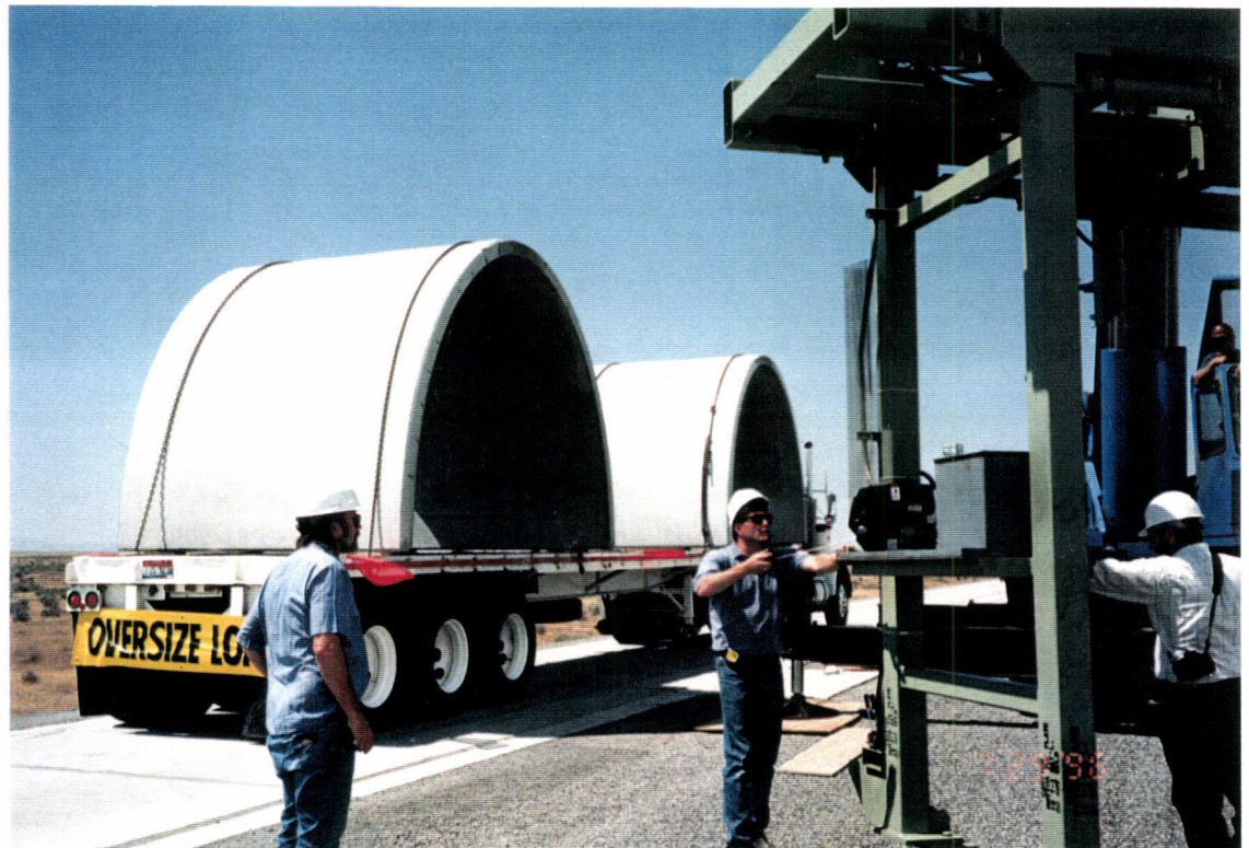
Another view of the type "C" beam tube enclosure module as they are delivered.
