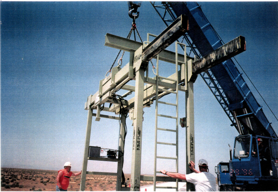
Crane is picking the beam tube enclosure lifting device.
