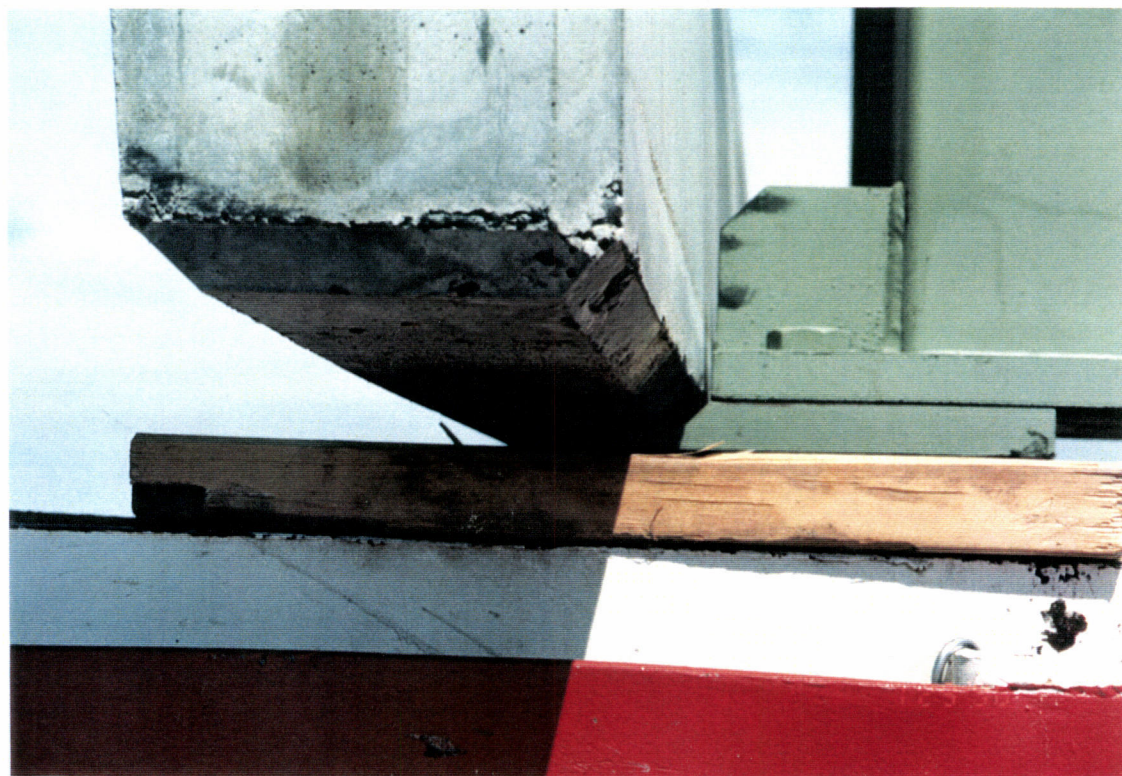
Close up view of the lifting foot as it is set under the beam tube enclosure units for lifting.
