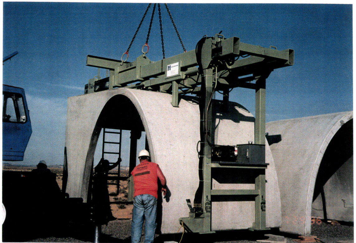
The type "A" beam tube enclosure module is set next to the type "C" modules in preparation for the mock up demonstration.
