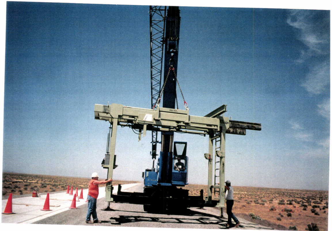
Crane is setting the lifting device in position for receiving the first type "C" beam tube enclosures.
