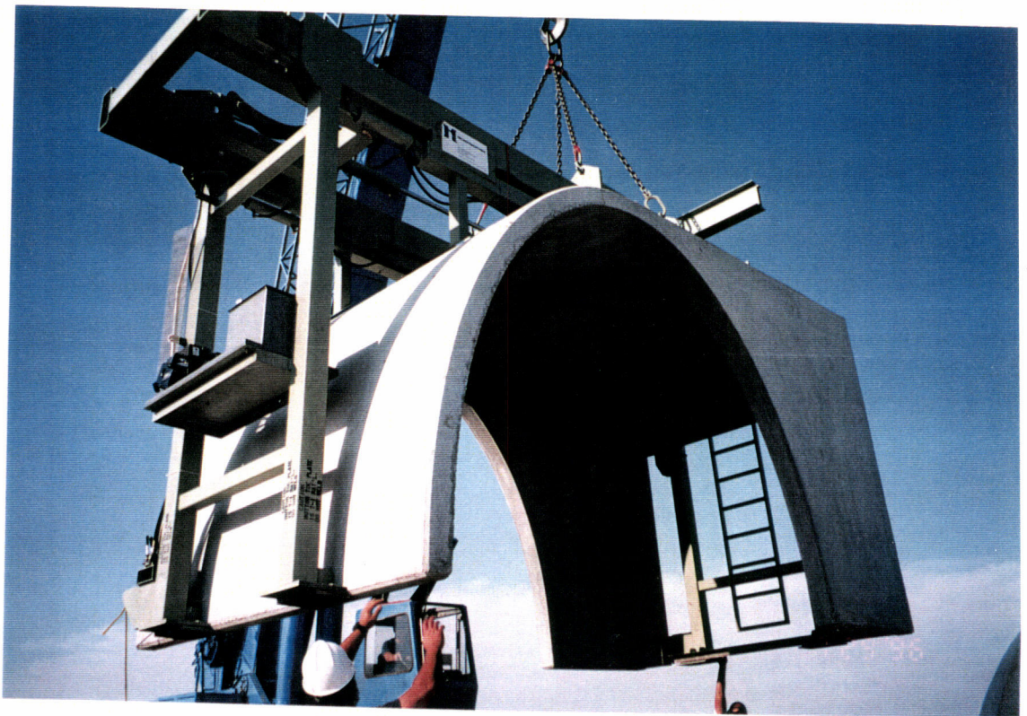
View of the unloading activities for the type "A" beam tube enclosure module.
