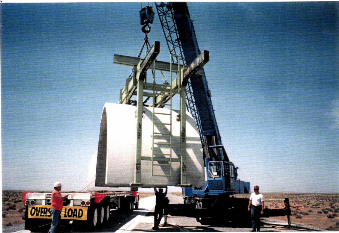
The first type "C" beam tube enclosure module is picked off the delivery truck.
