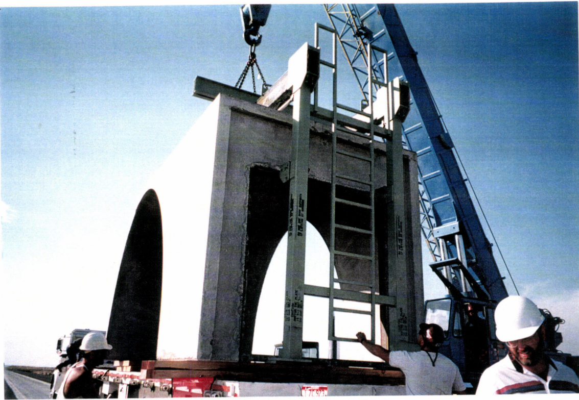
View of the unloading activities for the type "A" beam tube enclosure module.
