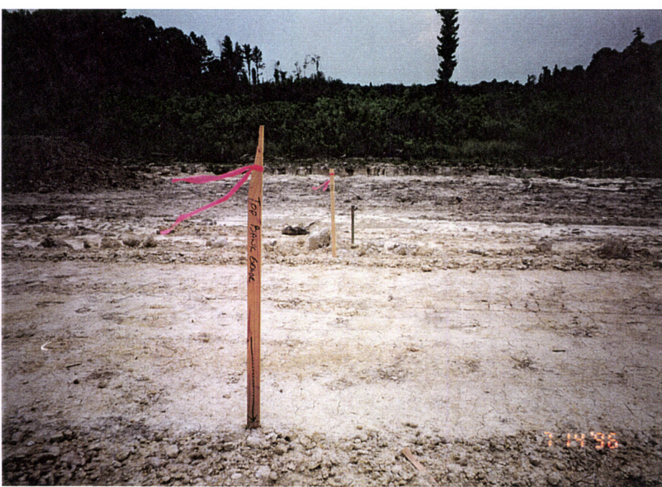
13. Grade stake at Sta. 68+00 on Southeast Arm. (Fill at finish grade).
