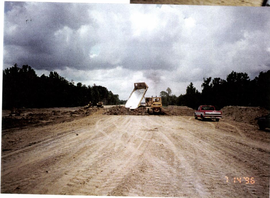
12. Dumping and spreading fill at Sta. 86+00 on Southeast Arm. (Looking North).
