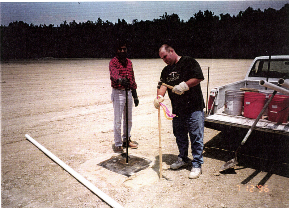
7. Installation of settlement monitoring plate at Corner Station.
