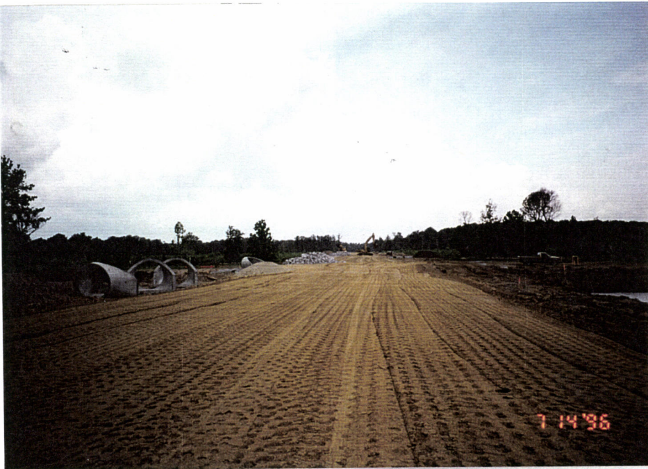
16. Fill compacted by sheepsfoot roller at Sta. 85+00 on Southwest Arm. (Looking West).
