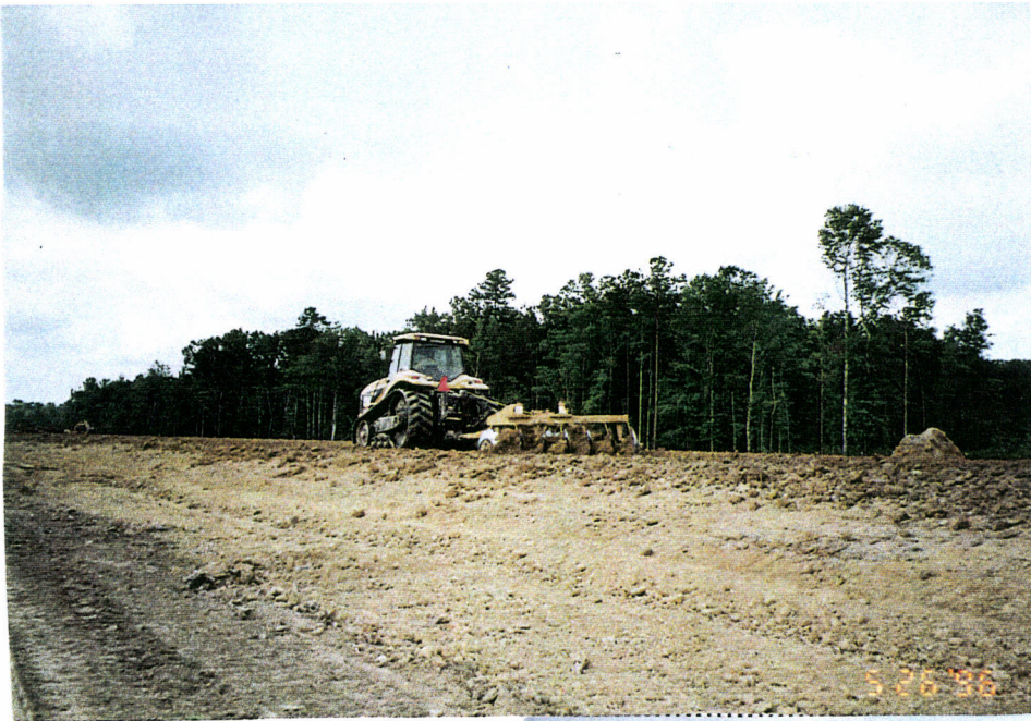
7. Southeast arm at station 70+00 disking berm lift.
