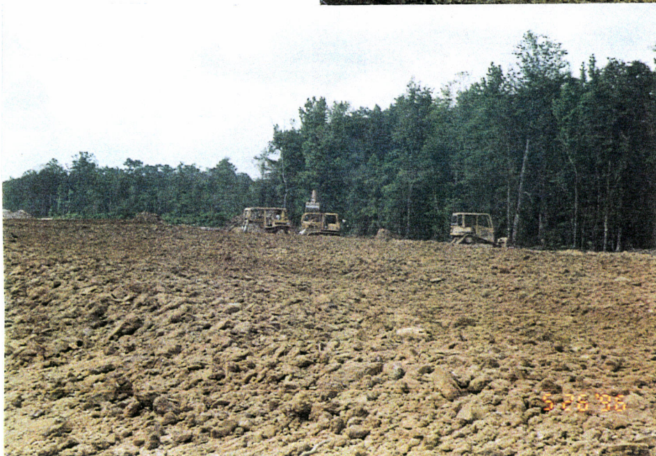
9. Southeast arm at station 17+00 , the first lift of berm.
