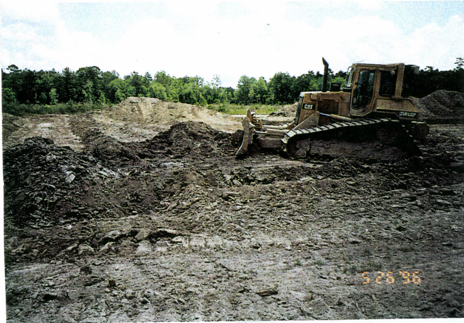
4. Southeast At station station 40+00 a dozer building berm.
