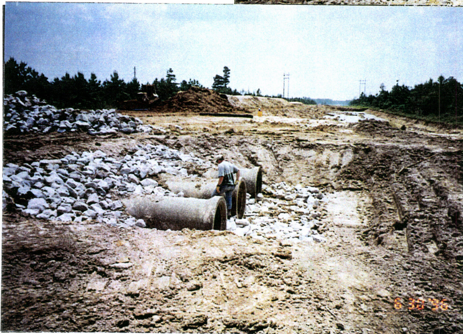
21. Southwest Arm looking West. Rip-rap being installed on 3'-36" dia. culverts at Sta. 60+00.
