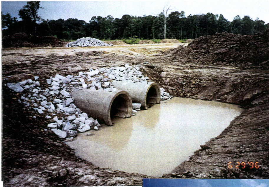
19. Southwest Arm looking Southwest. Rip-rap around culverts at Sta. 111+00.
