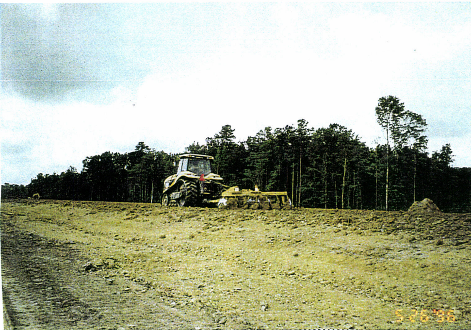
7. Southeast arm at station 70+00 disking berm lift.
