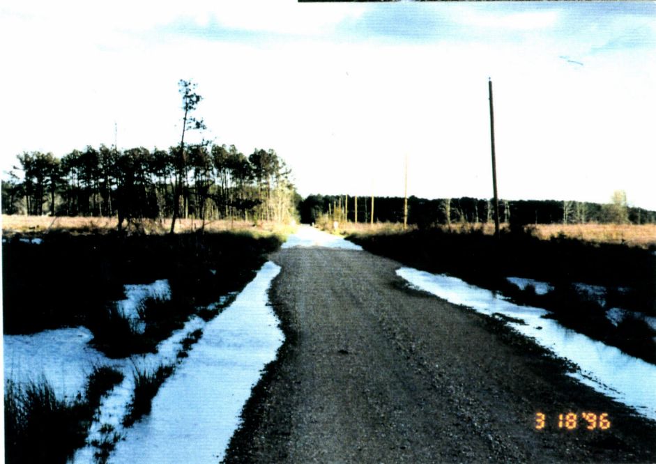
12. A close up view showing flooding of the road west of the cattlegaurd.
