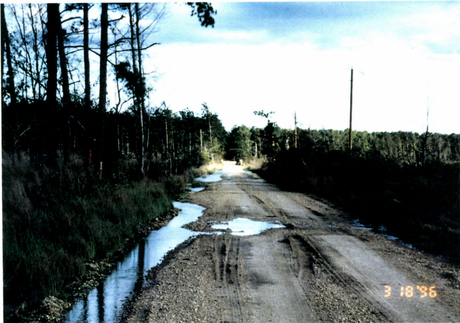
G960095-13-OP 13. This is the South entrance road to the end of the Southeast arm , showing flooding of road.
