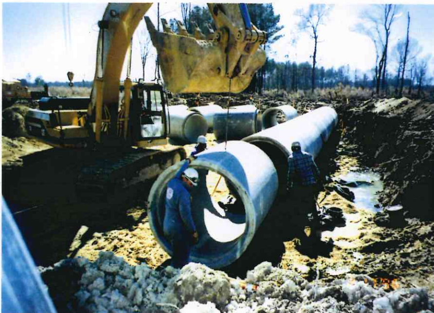
3. Installing 60" culvert pipe at crossing 44+60, Southwest arm.
