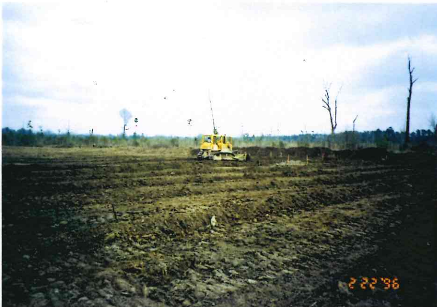
15. Southeast arm at station 112+00 dozing organic material to the side.
