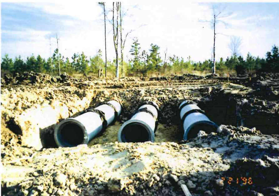
12. Southwest arm at station 60+00 showing cross section of backfill
