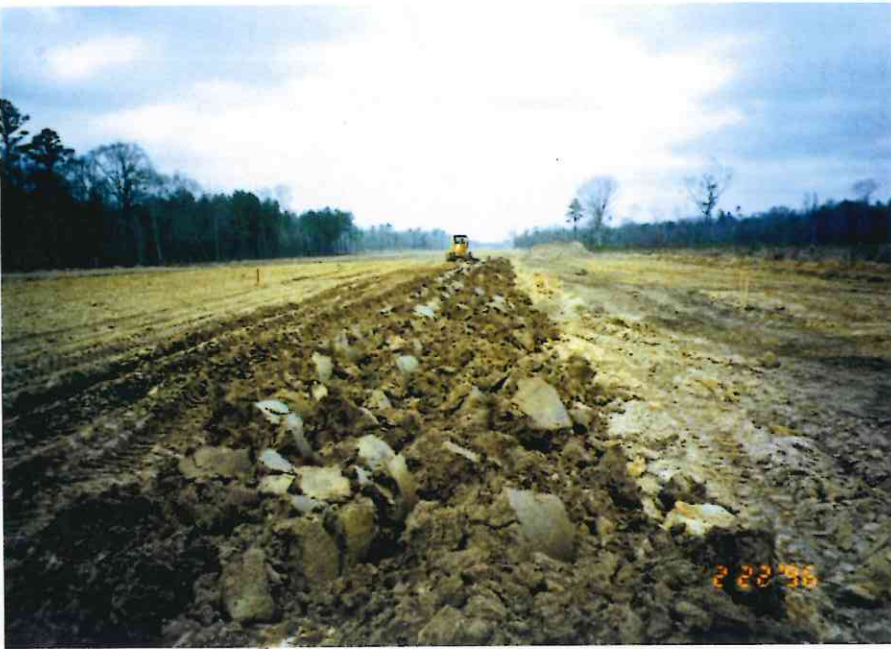
13. Southeast arm about station 113 looking north, disking berm
