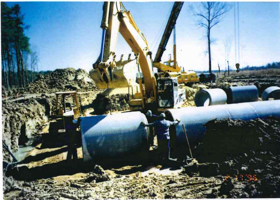
4. Southwest arm , at Station 60+00, installing 60" culvert pipe.
