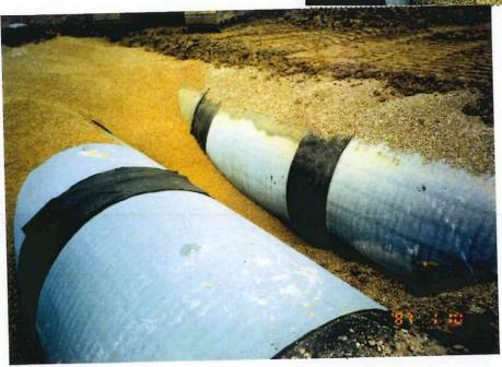
24.Southwest arm at station 123+00 culvert crossing backfil operation.
