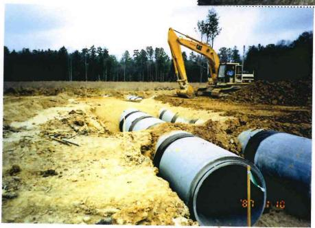
21Soutdhwest arm at station 123+00 culvert crossing. backfill operation
