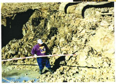
3.Southwest arm at station 16+40 excavating for culvert crossing.
