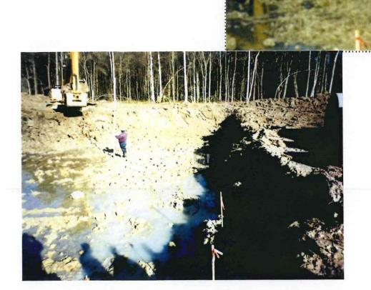
6 Southwest arm at station 16+40, checking grade at culvert crossing
