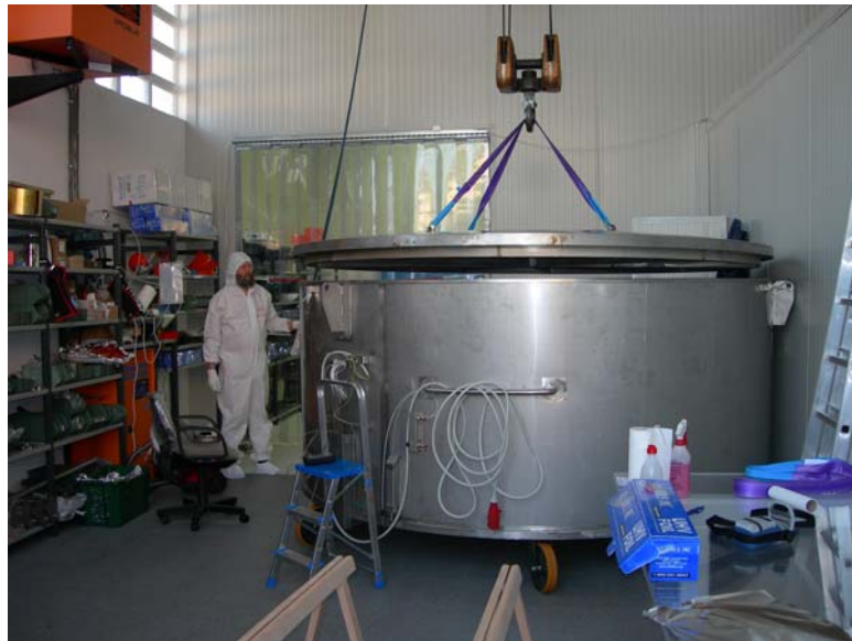
Large Air Bake Oven developed for Seismic Isolation Part Cleaning
