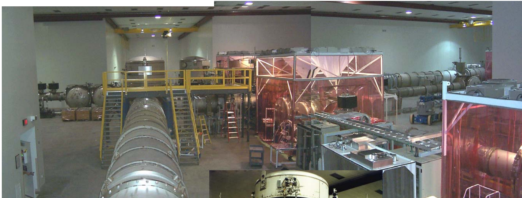
The view inside the Corner Station
