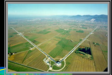
VIRGO: 3km Commissioning
