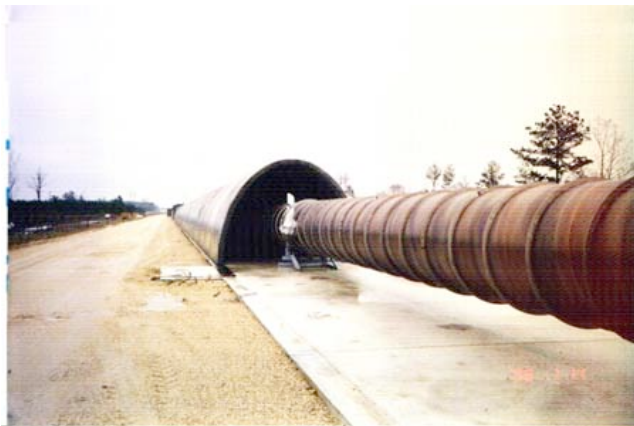
1.2 m diameter - 3mm stainless 50 km of weld NO LEAKS !!
