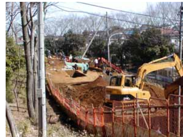
Construction around the site
