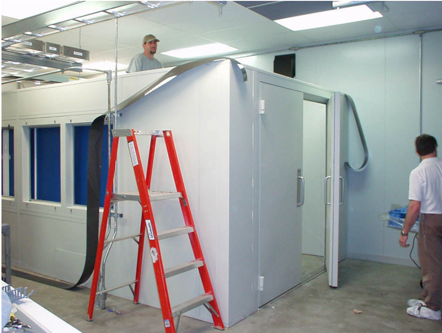
ENTRY DOORS – ACCESS OPENINGS WITHOUT THEIR COVERS.
