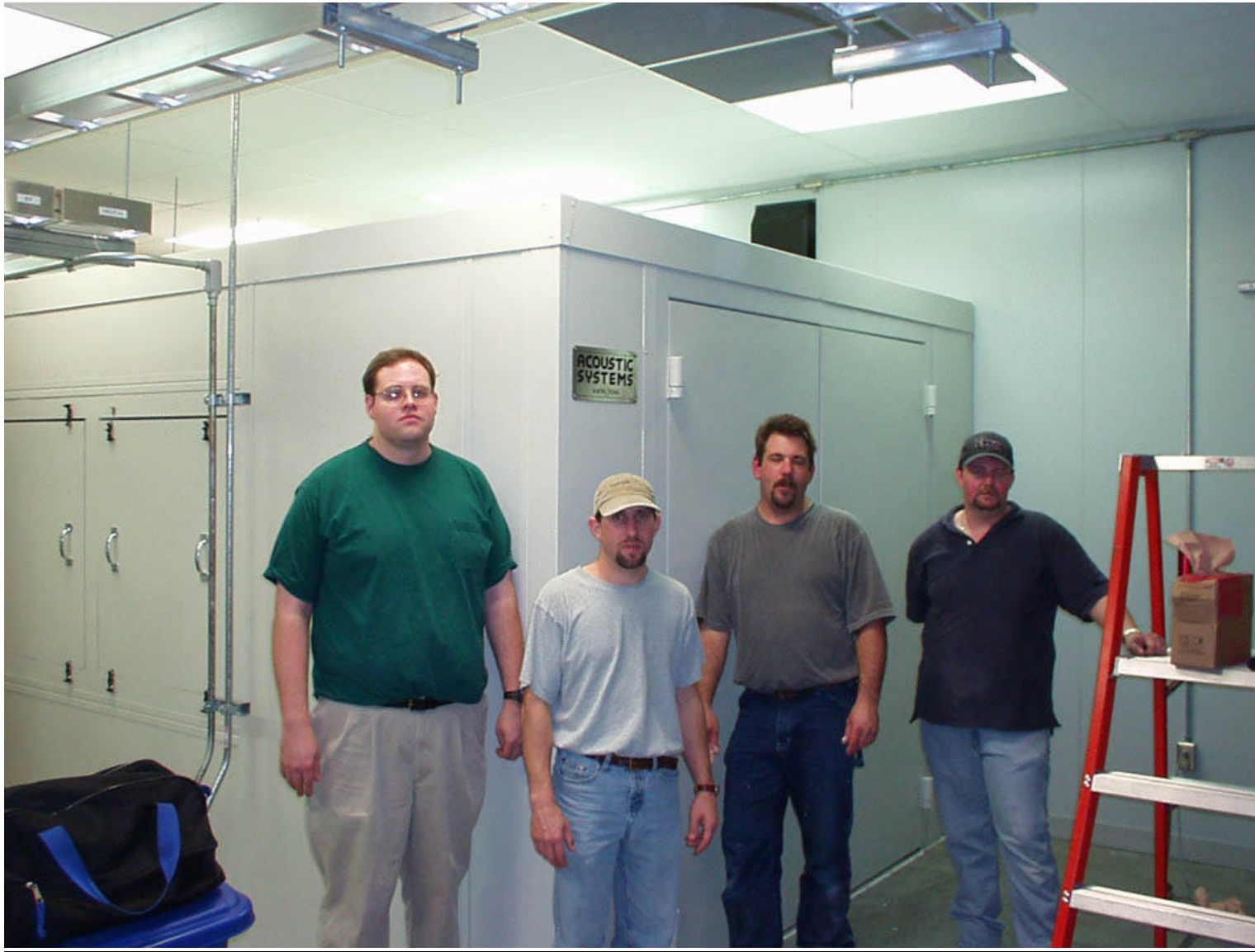
FINISHED INSTALLATION... Beer :30
