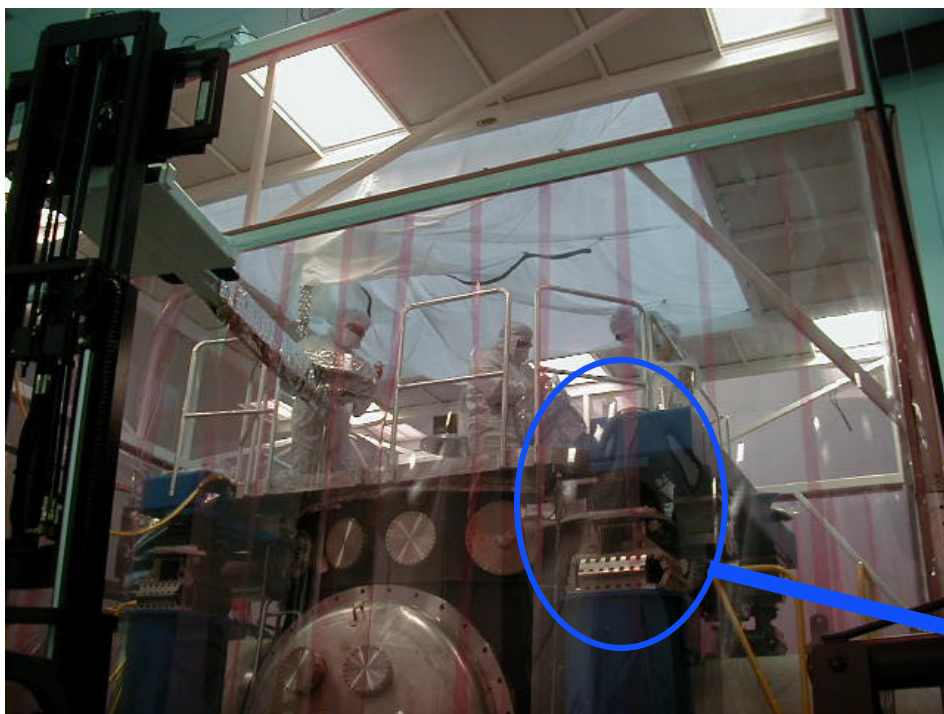
Stack Installation (Hanford X-Mid)
