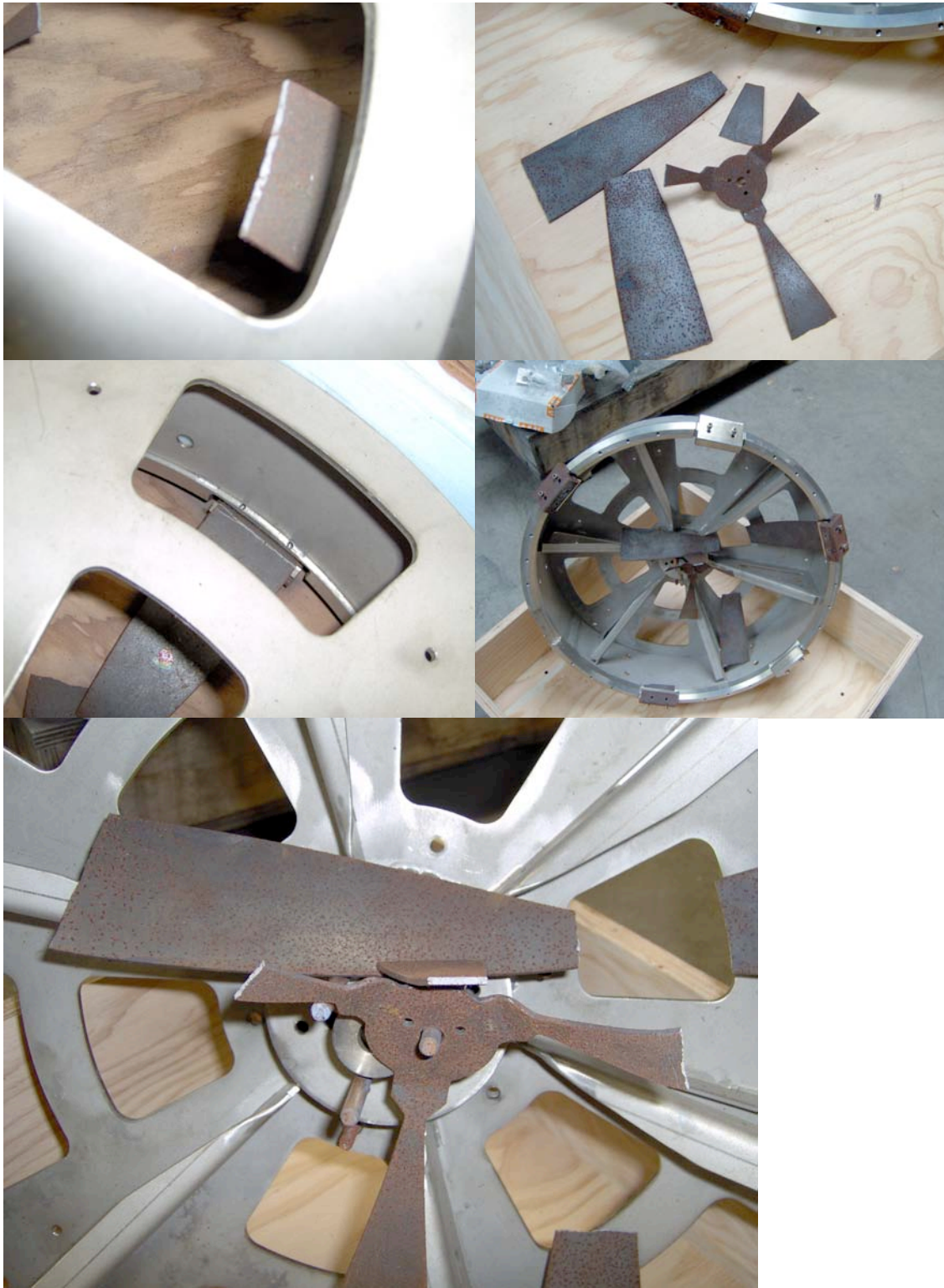
Figure 4, detail of the exploded blades, showing the effects of “classical” stress-corrosion.
