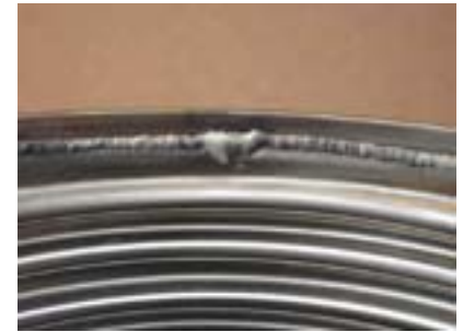
Suspect Weld 5.jpg
