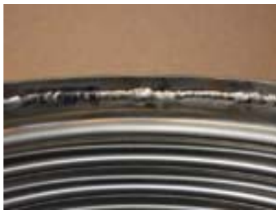
Suspect Weld 7.jpg
