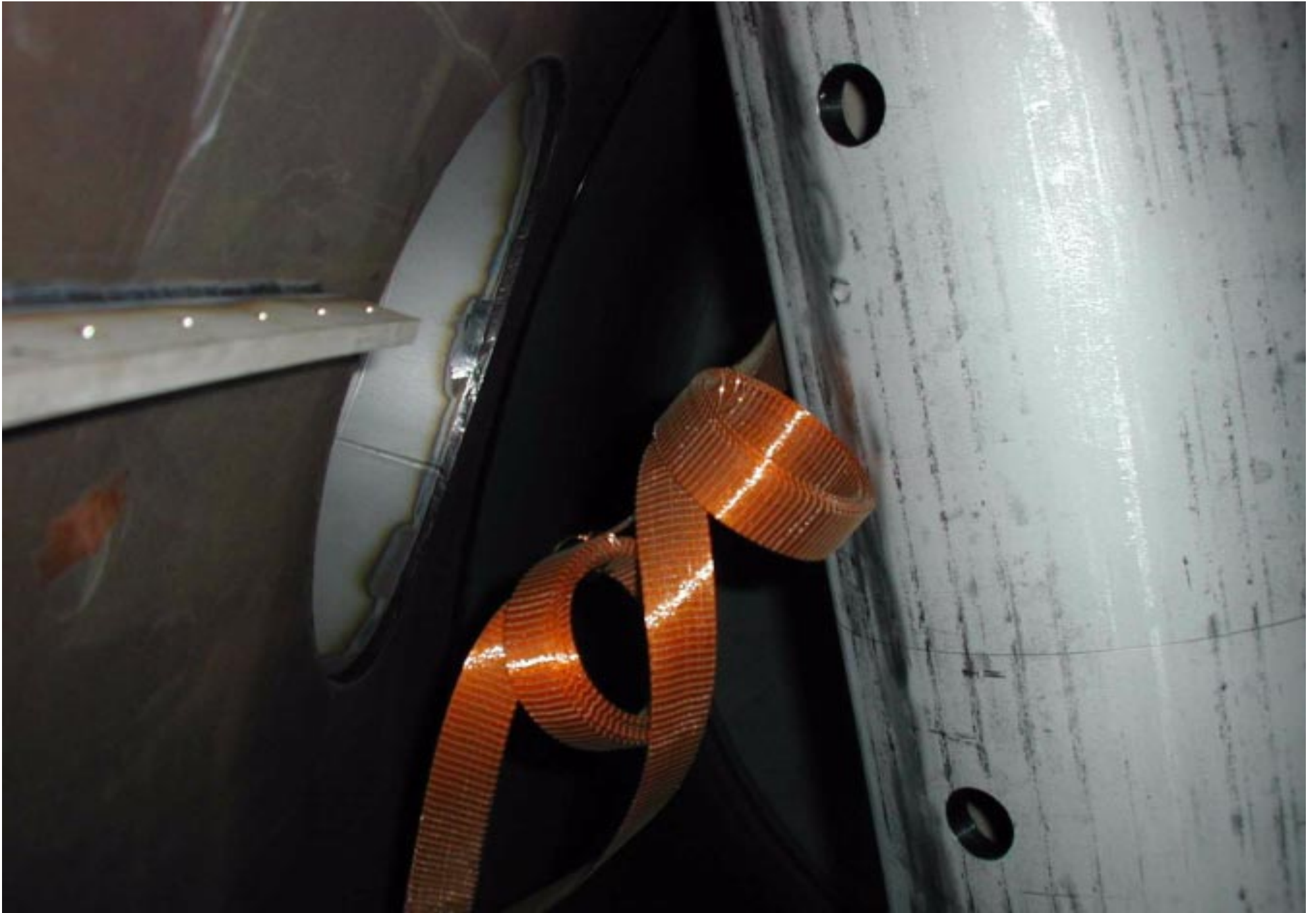
BSC 10 South Support Tube as viewed from below.
