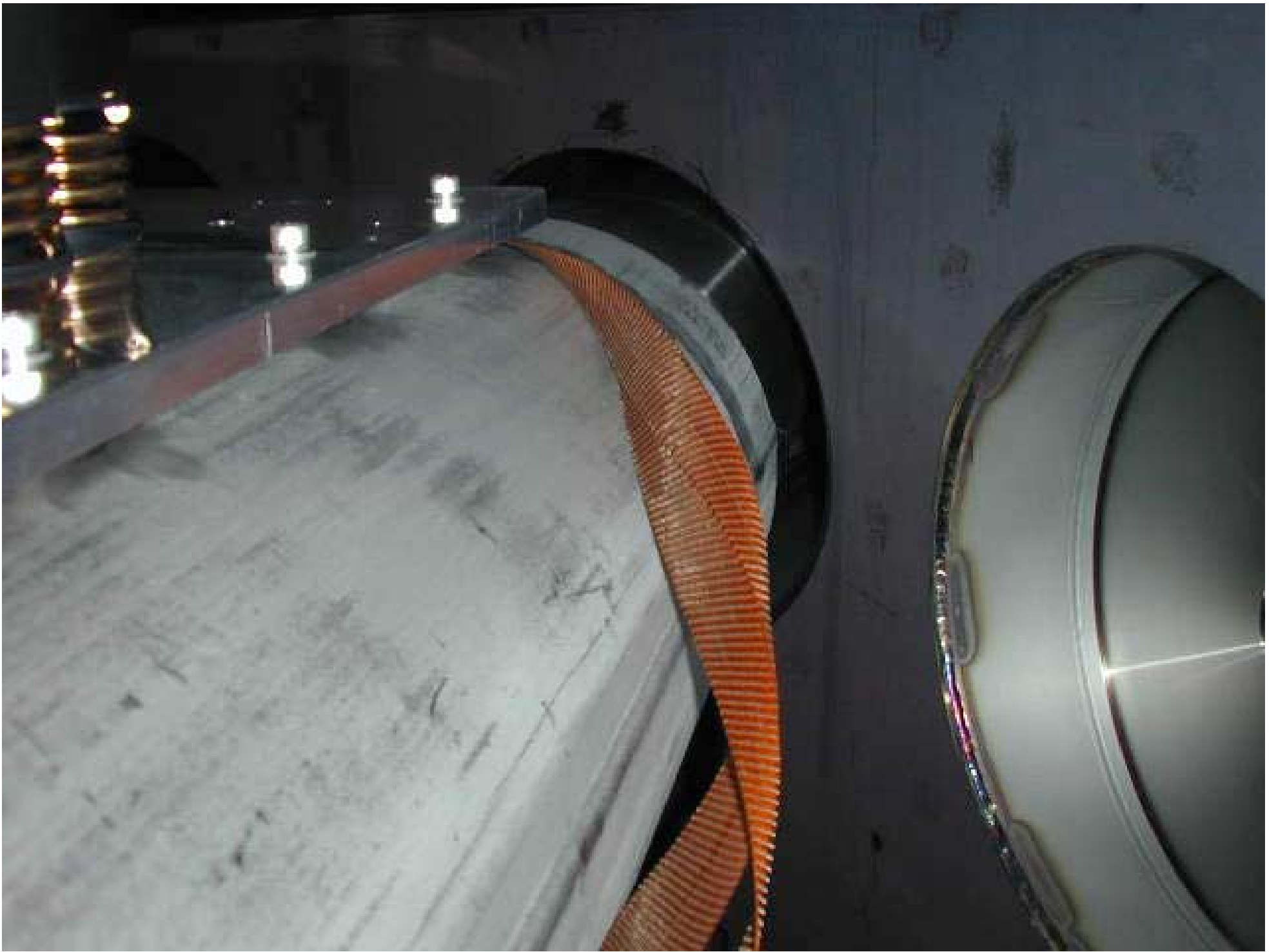
WBSC 7 May 12, 2000: 014. Cable tucked under NE corner, from E
