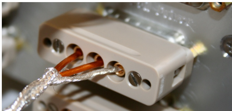
Figure – Actuator cable plugged on the feedthrough
