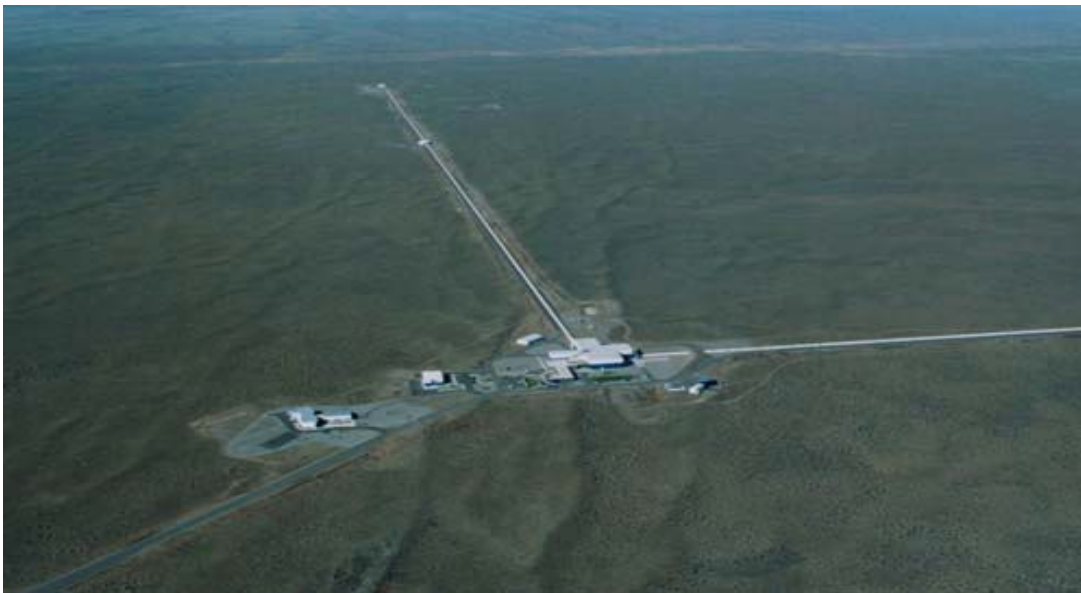
Figure 1: Aerial photograph of the LIGO Hanford Observatory. View is looking towards the SW, along the Y-arm. Two buildings are visible: one is at the 2 km midpoint; the other is at the 4 km terminus of the arm. The white structures along the arms are concrete covers protecting the vacuum tube.
