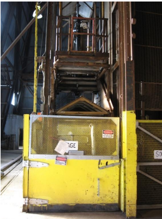
Figure 11: the Ross Shaft cage at surface level
