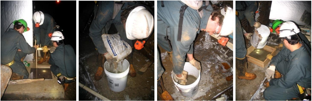
Figure 20,21,22,23: preparing the concrete plinth for the seismometer; in the center of figure 20 a granite tile is shown before it was placed on the concrete plinth inside the instrument hut
