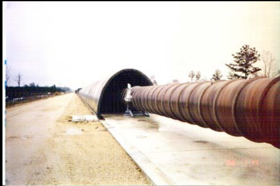
Evacuated Beam Tube
