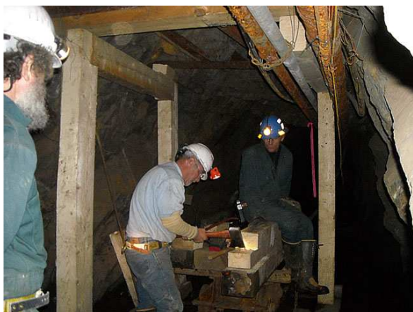
Figure 10: Supporting structure at the 800 ft level.
