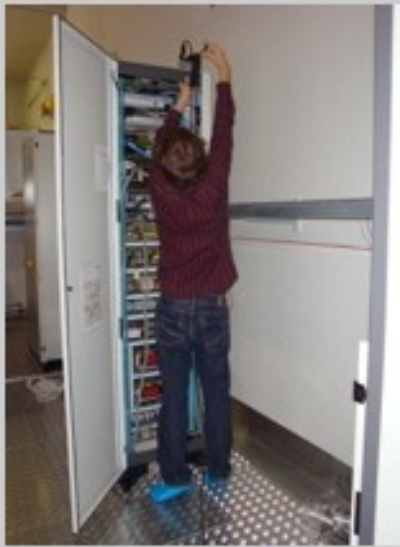
Casey installs accelerometers to measure fan noise directly
